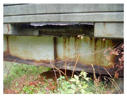
Figure 11. Deteriorated Deck Soffit and Beams: Route 99 Over Peak Creek
