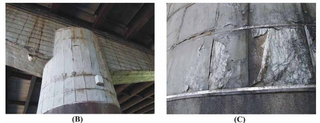
Figure 21. Zinc Foil Cathodic Protection System on Substructure of I-95 Over James River: (A) Series of Substructure Columns, (B) Typical View of Column And Bent, (C) Close-Up Showing Metal Loss and Peeling of Foil
