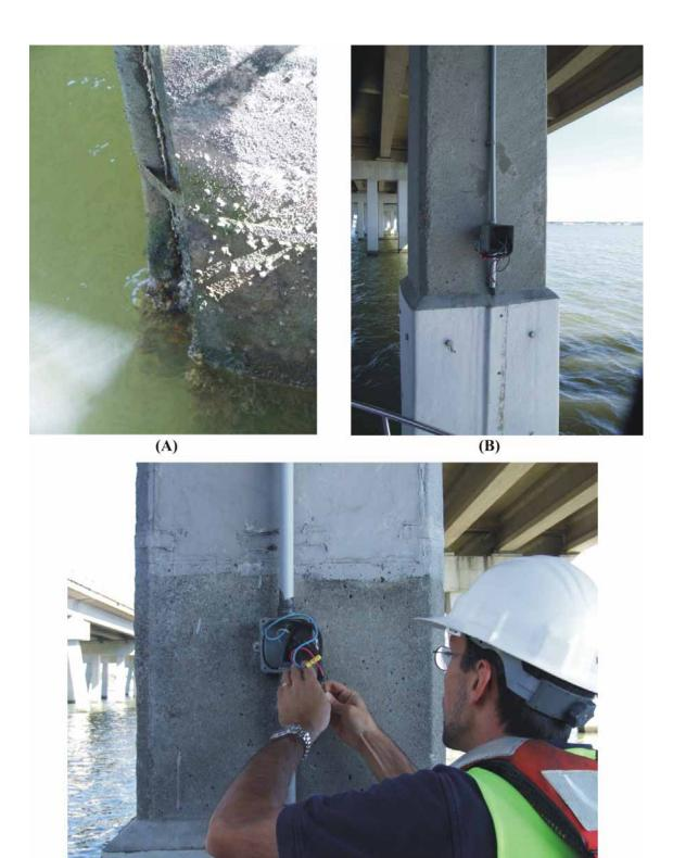
(C) Figure 5. I-64 EBL Over Willoughby Bay Substructure: (A) No Evidence of Sea Life Build-up Under Compression Panel, (B) Close-up of Structural Jacket Containing Galvanic Cathodic Protection System, (C) Zinc Hydrogel Anode (Upper Pile Region) in Contact with Concrete Surface and All Conduit in Place and Watertight
