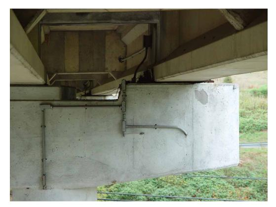
Figure 16. Conductive Coating Cathodic Protection System on Substructure of I-81 SBL Over Mill Creek
