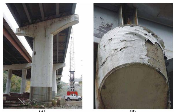
(A) (B) Figure 18. (A) Substructure Cathodic Protection Coating System with (B) Coating Adhesion Loss on I-81 NBL Over Maury River
