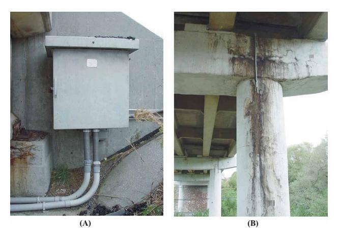
Figure 17. (A) Control Unit and (B) Deteriorated Cathodic Protection Coating on Piers of I-81 SBL Over Mill Creek
