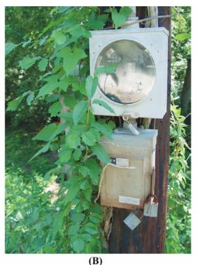
Figure 14. (A) Control Unit and (B) Locked Out Power Meter for Decommissioned Cathodic Protection Deck System: Route 15 Over Willis River
