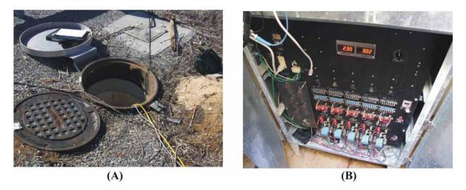
Figure 9. Impressed Current Cathodic Protection (ICCP) Rectifier System Located in Control Bunker of Smart Road Bridge Over Route 642: (A) Open Bunker Access, (B) Control Panel for 5-Zone ICCP System (Note Missing Fuse for Zone 3) Shows Voltage and Current Display (with Switch on Zone 5)
