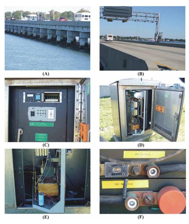
Figure 2. Inactive Cathodic Protection System on I-64 WBL Hampton Roads Bridge-Tunnel: (A) Overview of Hampton Roads Bridge, (B) Bridge Deck Surface, (C) Face of Cathodic Protection Rectifier, (D) View Inside Electronics Cabinet, (E and F) Close-up of Electrical Components
