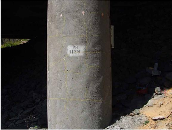
Figure 24. Highlighted Shrinkage Cracks (visible as light lines in grid pattern) in Column P12: Route 29/Route 250 Over Route 654
