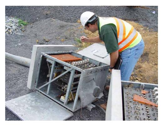
Figure 19. Inspecting Decommissioned Cathodic Protection Control Units: I-81 NBL Over Maury River
