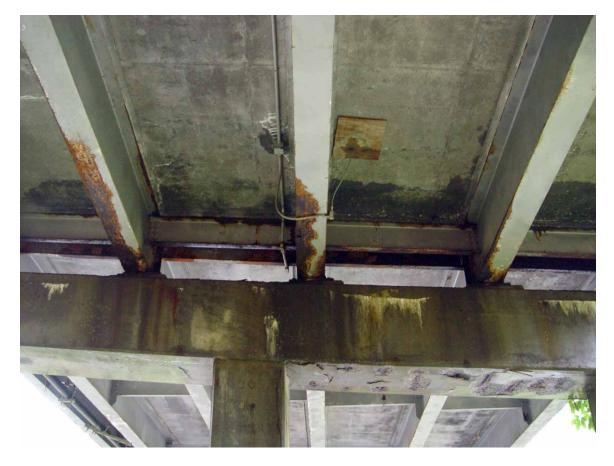
Figure 12. Underside of Deck with Cathodic Protection System Connections: Route 99 Over Peak Creek
