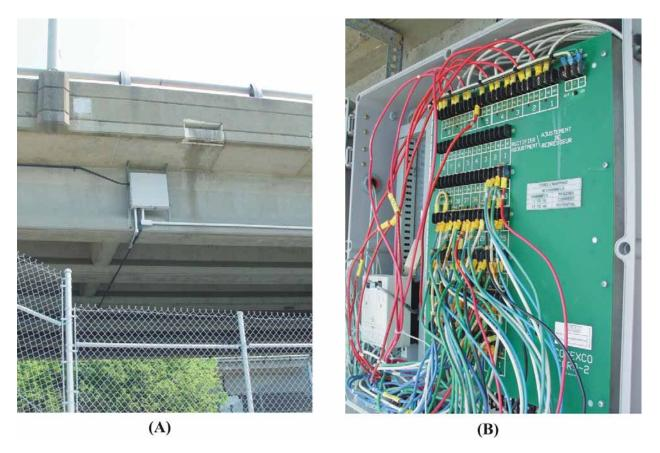
Figure 4. Control Unit for Substructure Cathodic Protection Systems: I-64 Over Willoughby Bay
