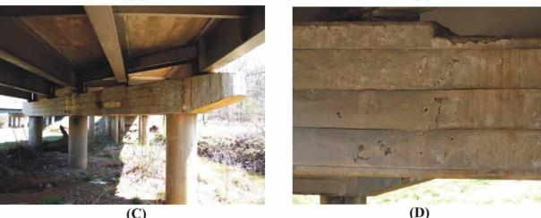
Figure 25. Conductive Coating on Substructure: Route 58 EBL Over Leatherwood Creek
