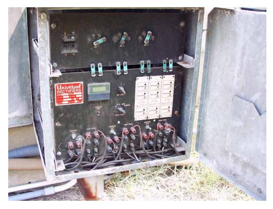
Figure 6. Control Unit for Cathodic Protection System: I-64 EBL Over 13th View Street
