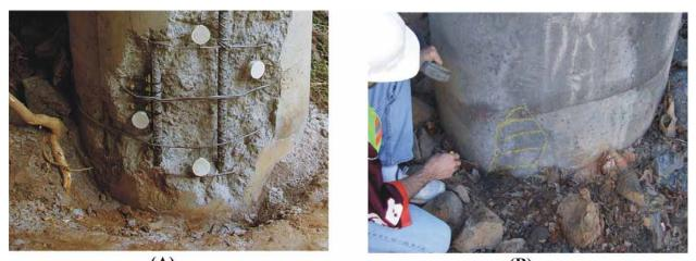
(A) (B) Figure 23. Column P1 (A) Prior to Shotcrete and (B) with Subsequent Delamination (hatched area): Route 29/Route 250 Over Route 654
