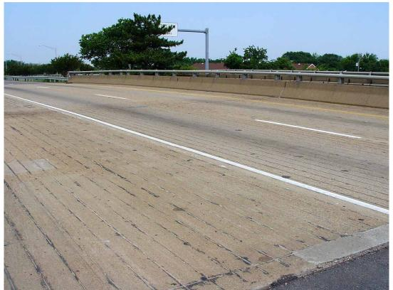
Figure 7. Cathodic Protection System on Deck of I-64 EBL Bridge Over 13th View Street
