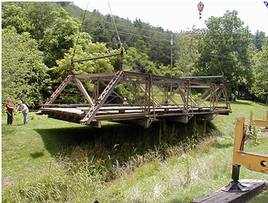
Figure 43. Moving Pony Truss Bridge
