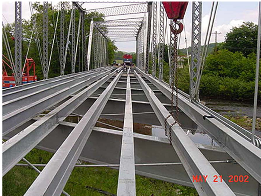
Figure 34. Installation of Stringers
