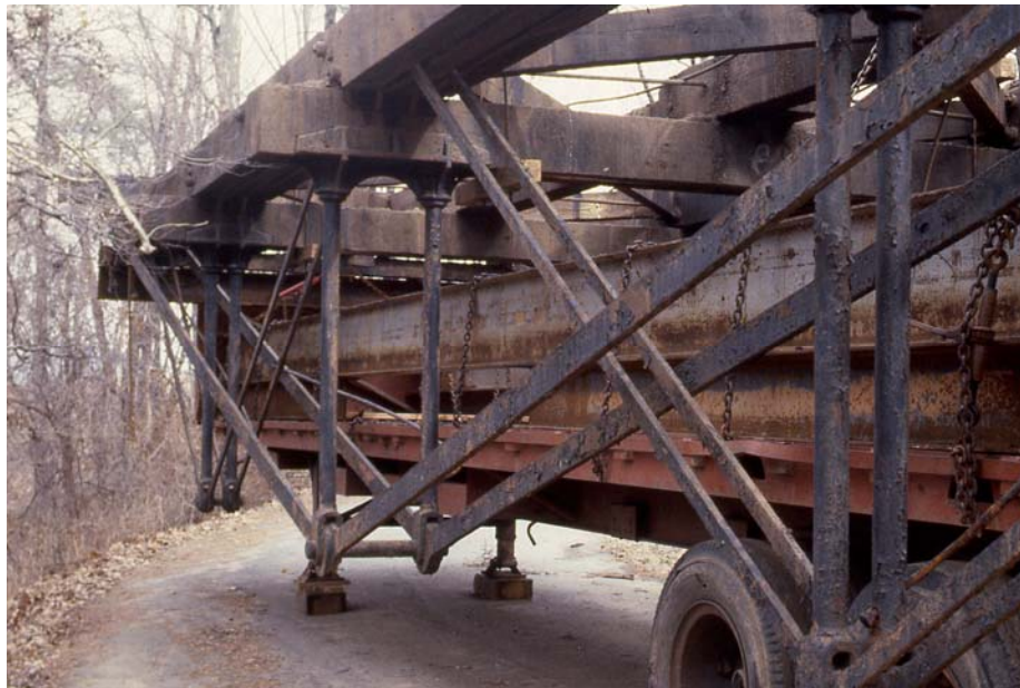
Figure 39. Moving Fink Truss
