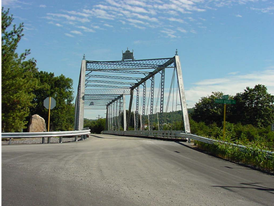
Figure 37. Rehabilitated Goshen Bridge, 2002
