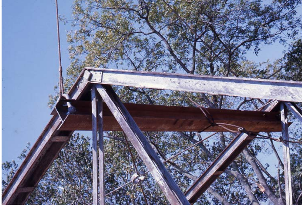
Figure 42. Lifting Apparatus at Hip Joint, 106-foot Truss
