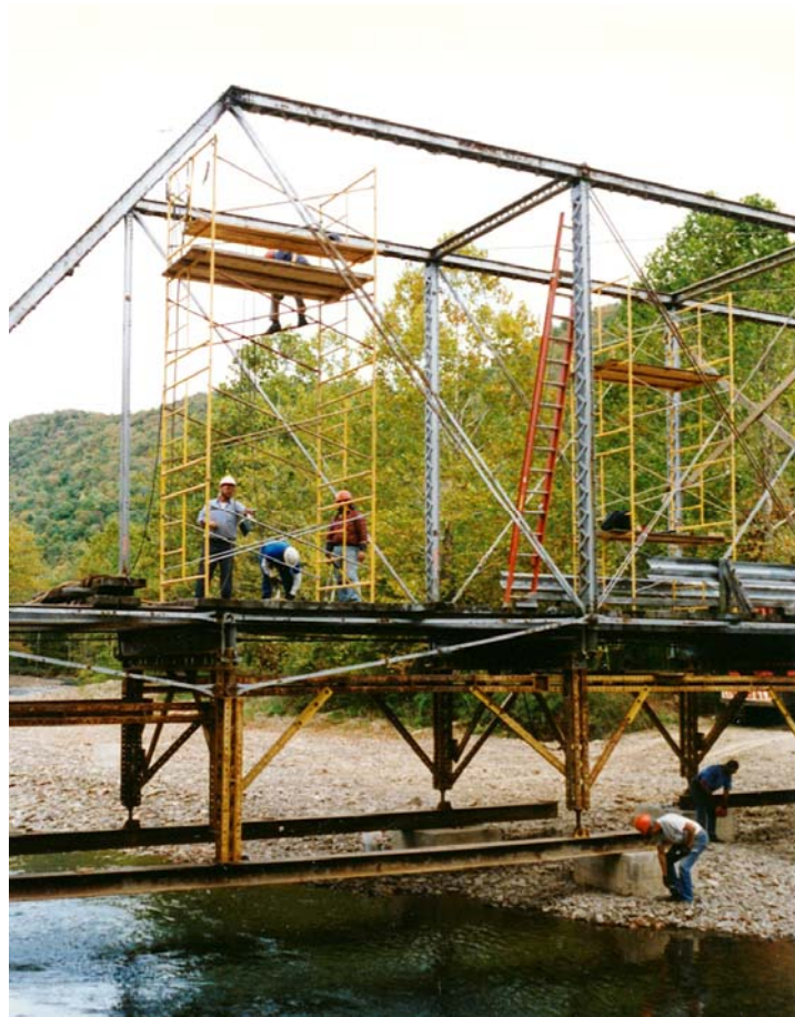
Figure 8. Falsework System Supporting Each Panel Point
