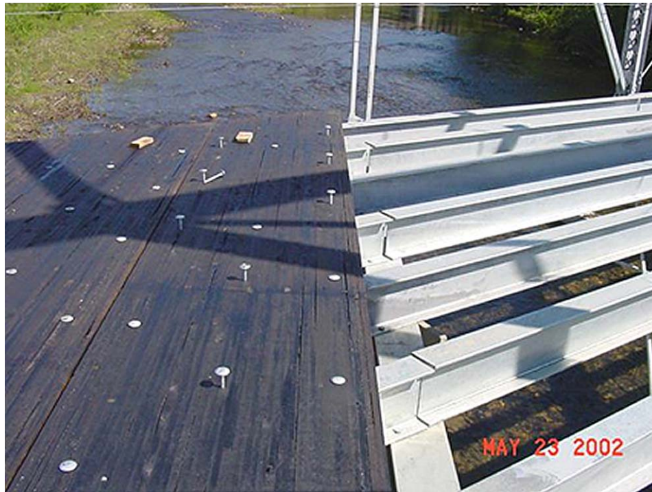
Figure 35. Glued Laminated Timber Panel Installation
