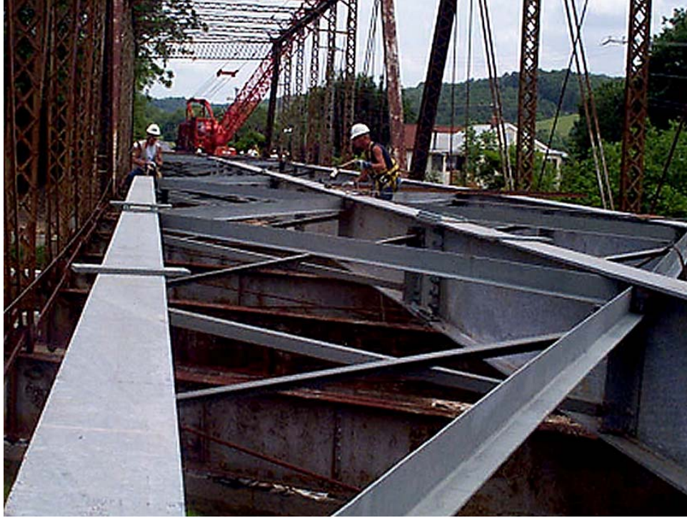
Figure 6. Falsework Beams during Installation
