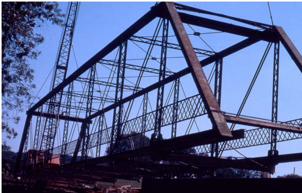
Figure 41. Lifting 106-foot Pratt Truss
