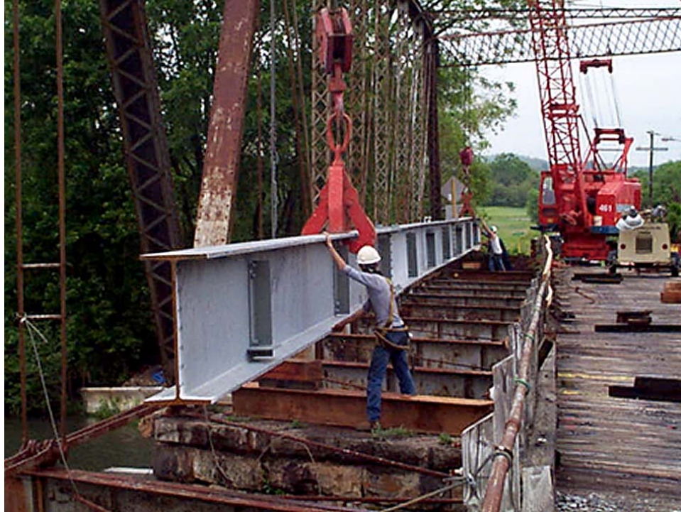
Figure 24. Placing Falsework Beam
