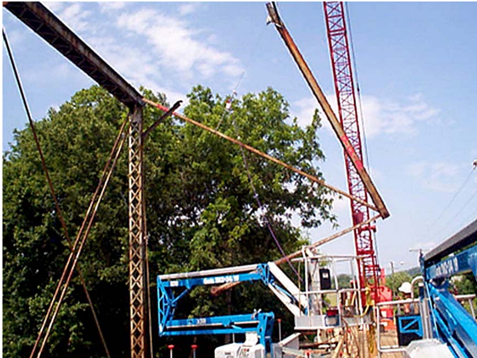
Figure 28. Cranes Remove Sections of Truss
