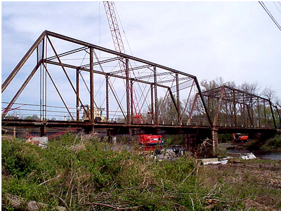
Figure 1. Route 746 Bridge Over Calfpasture River at Goshen, Virginia
