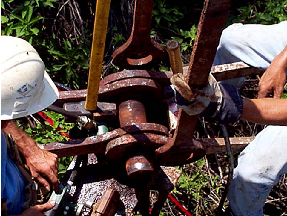
Figure 25. Jacking Truss Members Apart on Goshen Bridge
