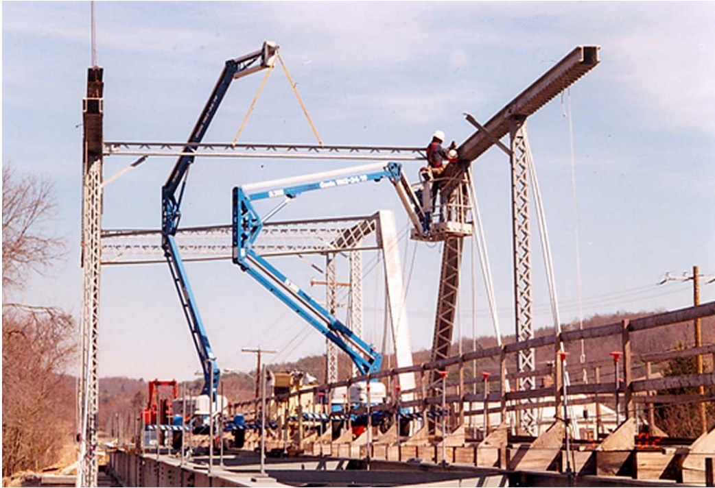
Figure 22. Light Electric Lifts During Re-Erection of Truss
