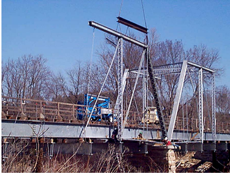
Figure 32. Re-erection of Trusses
