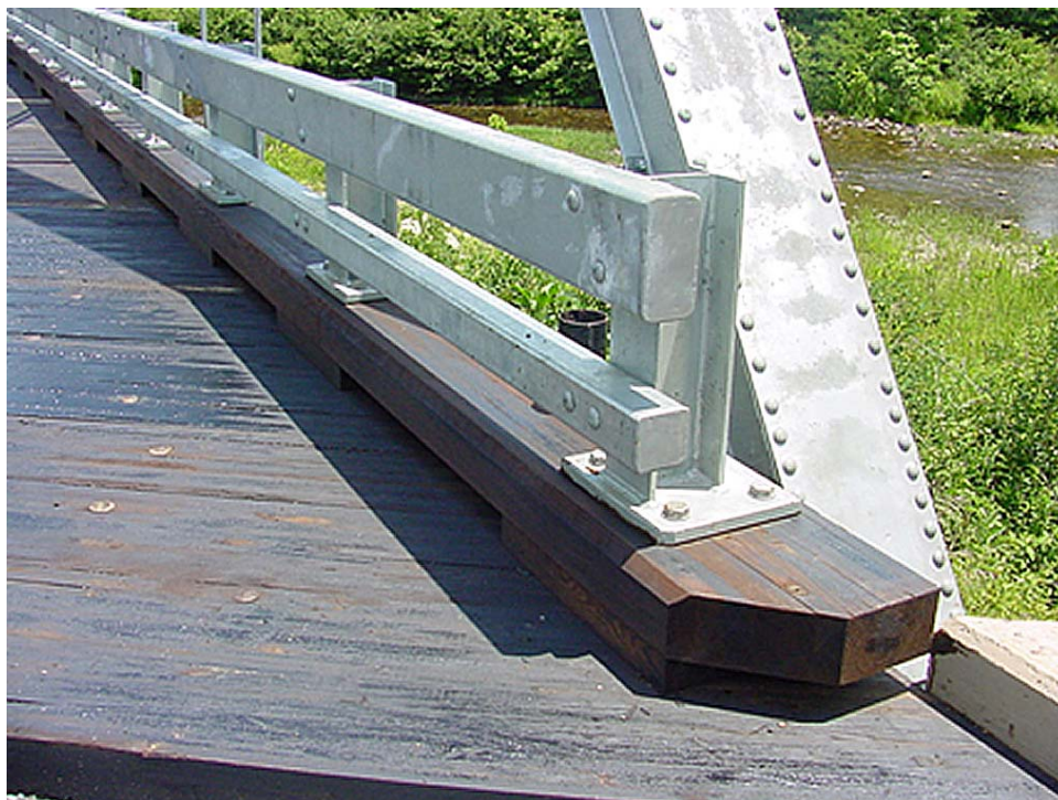
Figure 36. Modified Illinois Rail Protects Truss
