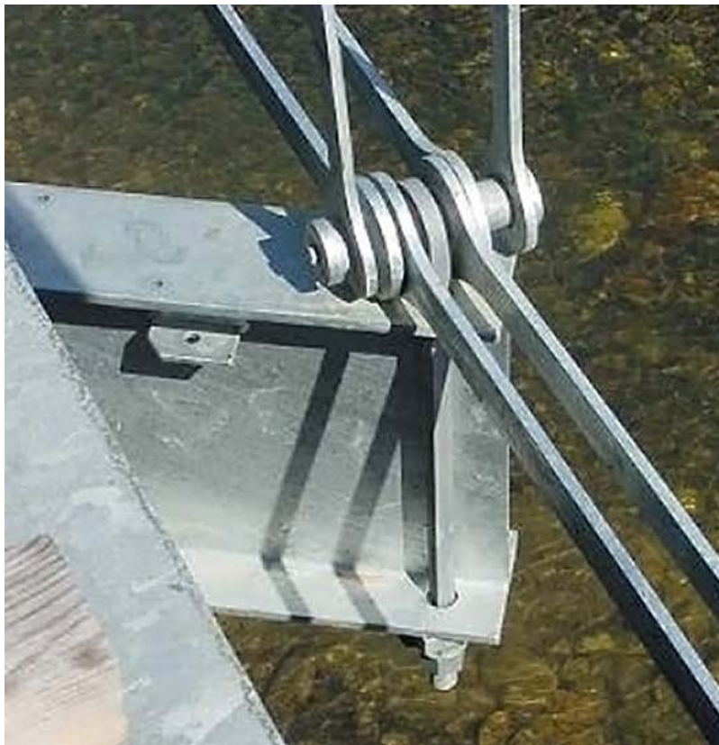
Figure 20. Final Truss Member Assembly at Lower Panel Point
