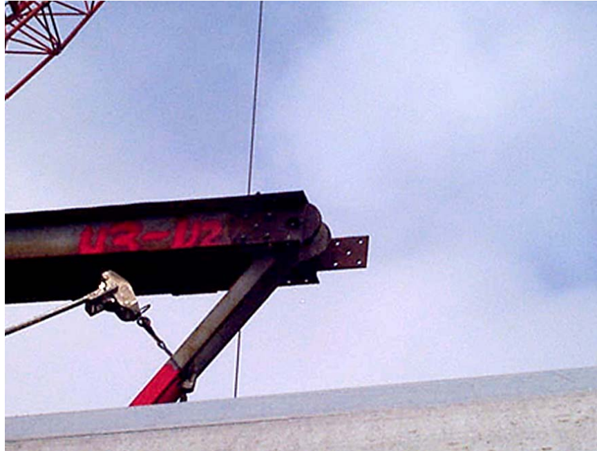
Figure 29. Supporting Diagonal After Pin Removal
