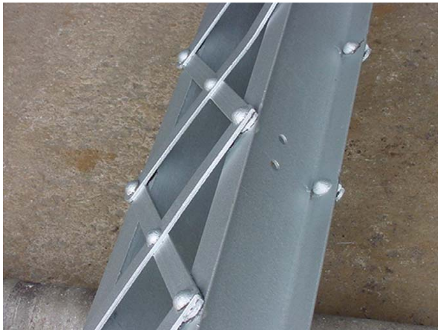
Figure 30. Original Vertical Member After Cleaning and Galvanizing
