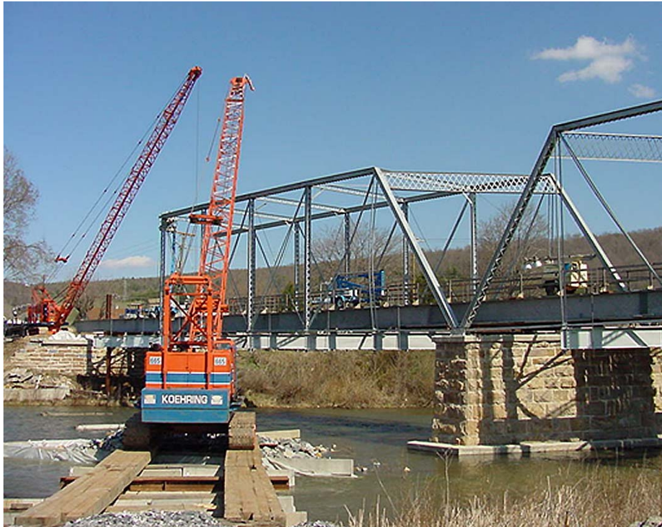
Figure 21. Crane Locations During Re-erection of Trusses
