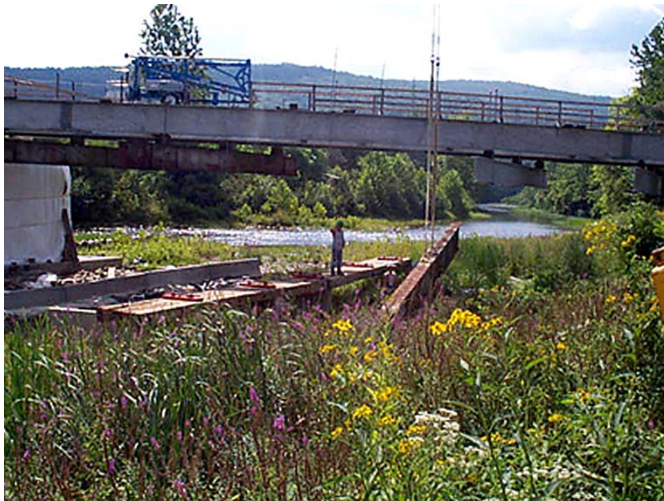
Figure 31. Floor Beam Replacement
