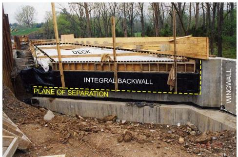
Figure 7. View of Completed Deck and Backwall
