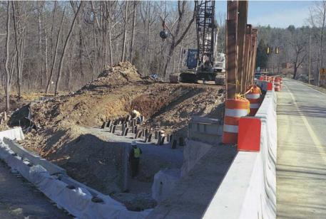
Figure 4. Foundation Piles at Abutment B
