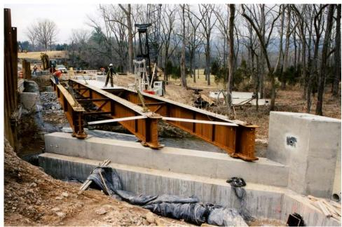
Figure 6. Placement of Structural Steel
