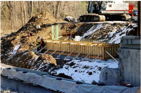
Figure 5. Formwork for Abutment B
