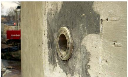
Figure 12. Load Cell at Abutment B
