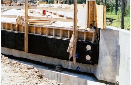
Figure 13. Earth Pressure Cells at Abutment B
