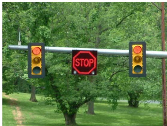
Figure 76. LED stop sign visual warning. Unlit strobes can be seen at the two bottom corners.
