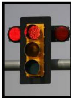
Figure 28. Dual flashing red lights.
