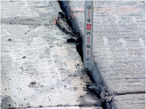
Figure 1. Differential Slab Movement at Longitudinal Joint
