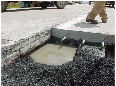
Figure 10. Trapped Water After Rain storm During Slab Replacement
