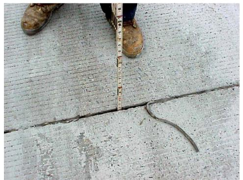
Figure 2. Broken Sealant at Transverse Joint
