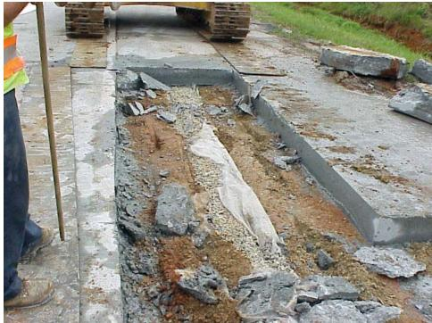
Figure 11. Discontinuity of Drainage Layer Under Shoulder Slab
