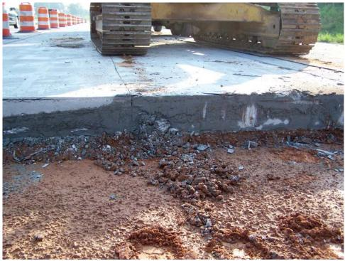
Figure 9. Soft Condition of Soil Cement Underneath Concrete Slab
