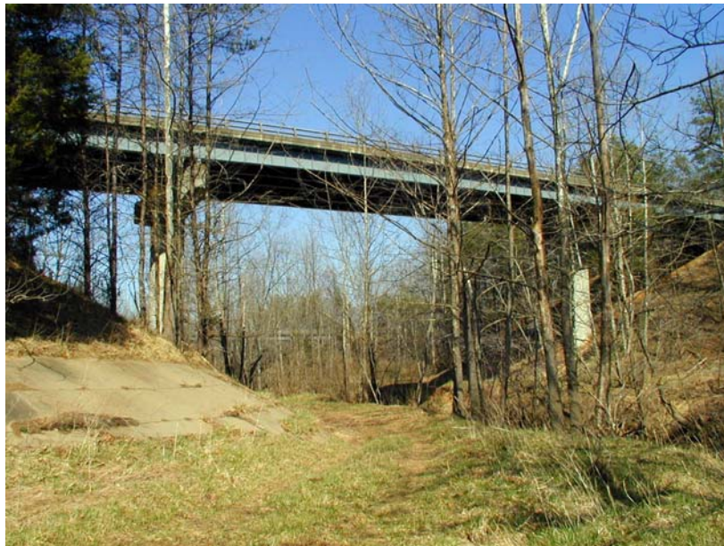
Figure 4. Site 2: Eastbound Bridge on I-64 West of Charlottesville
