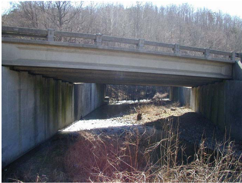
Figure 8. Site 6: Bridge Along I-81 North of Buchanan
