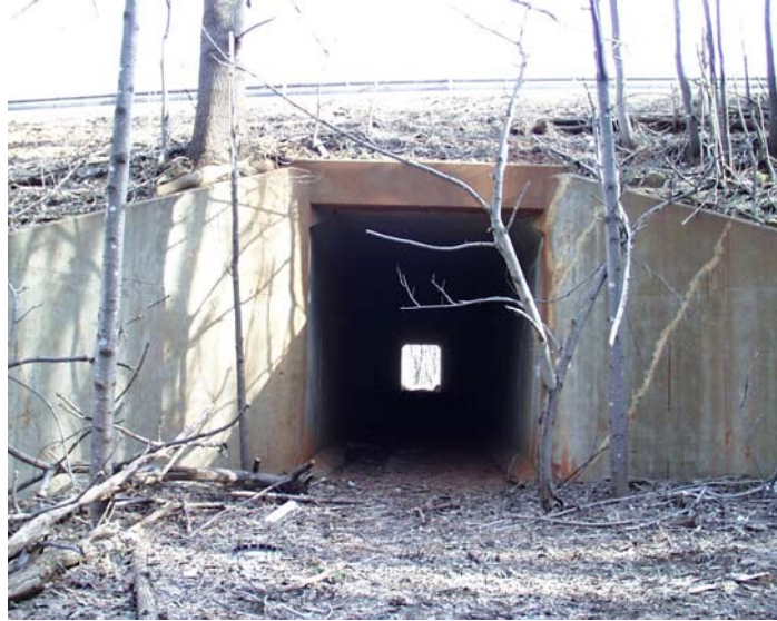
Figure 3. Site 1: Single-barrel Box Culvert West of Charlottesville
