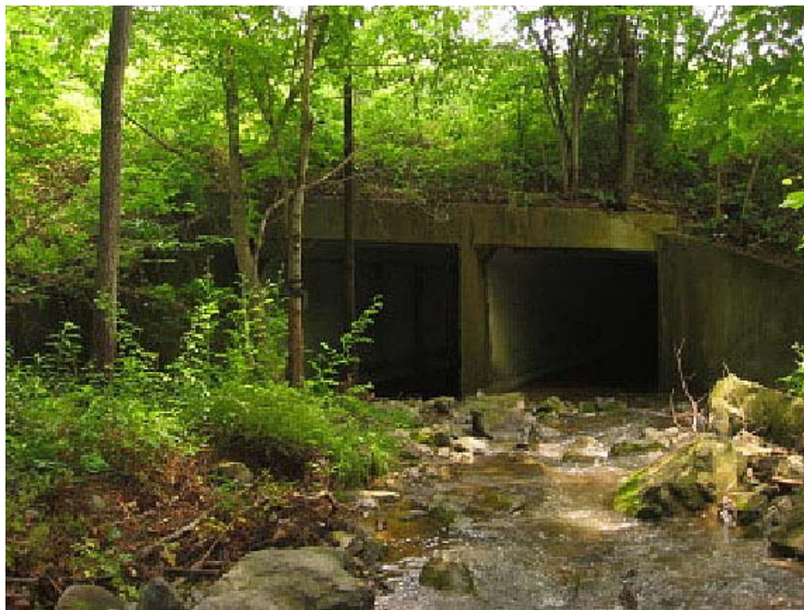
Figure 7. Site 5: Double-box Culvert Beneath I-81 North of Buchanan
