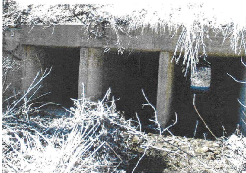
Figure 6. Site 4: Triple-box Culvert Beneath Route 340 North of Grottoes
