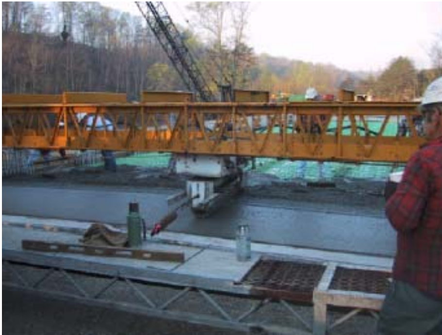
Figure 6. Span C Concrete Casting
