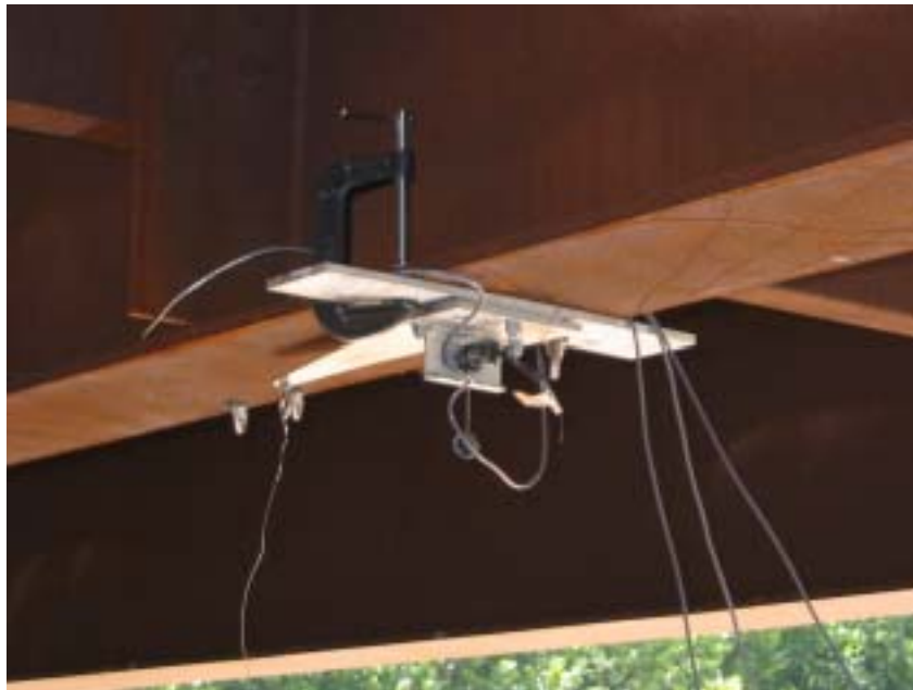
Figure 9. Deflectometer Clamped to Steel Girder
