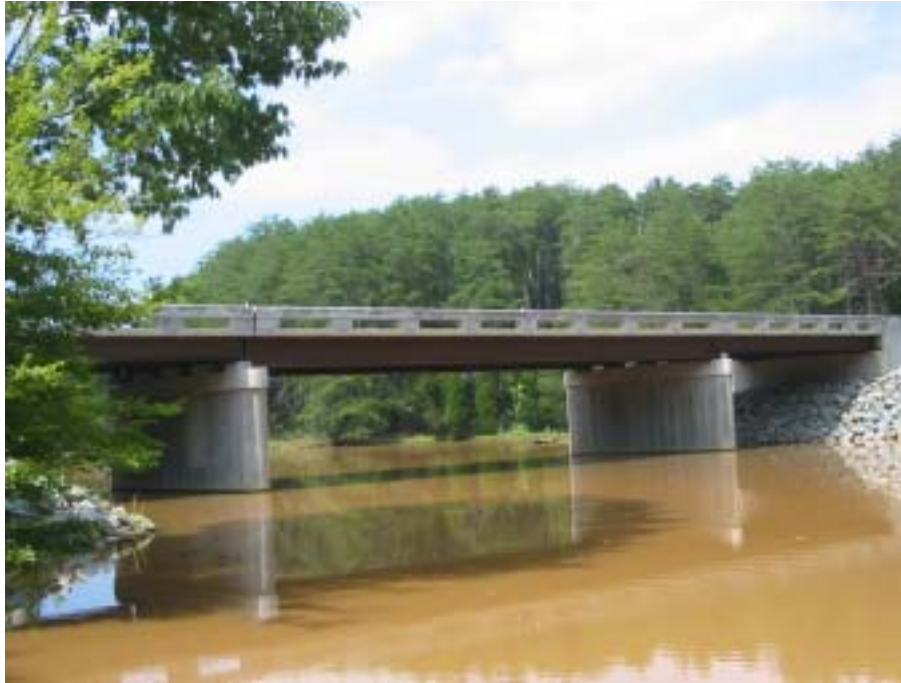
Figure 1. Route 668 Bridge Over Gills Creek
