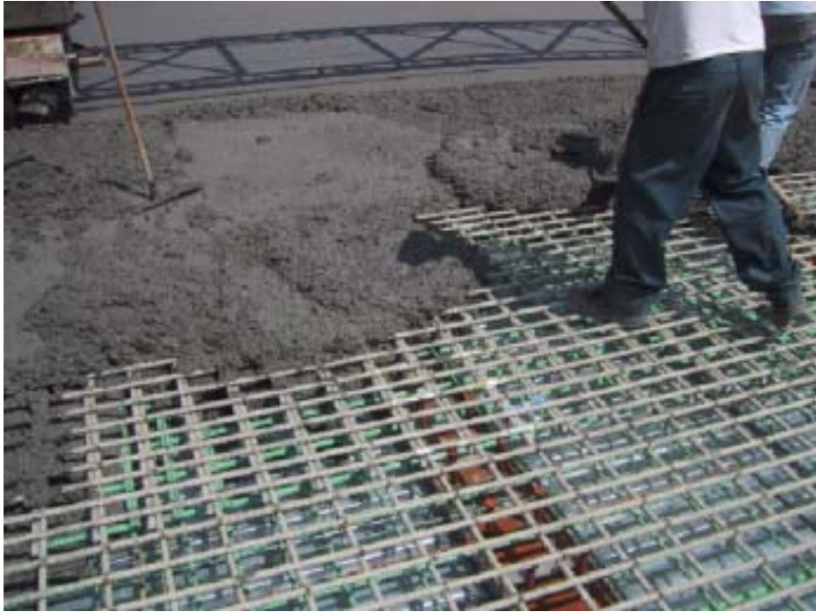
Figure 7. Span A Concrete Casting
