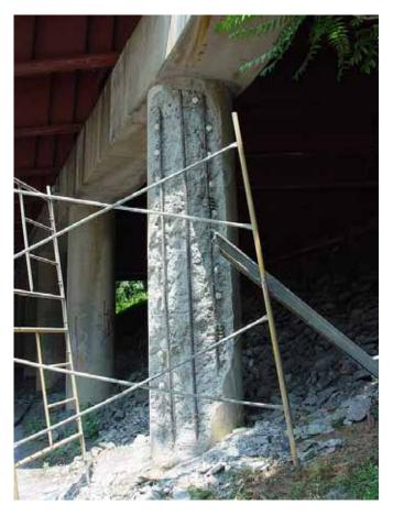
Figure 3. Placement of Anodes in Shotcrete Repair Areas
