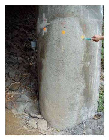
Figure 4. Electrical Potential and Resistivity Test Locations After Repair
