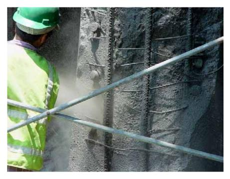
Figure 9. Placement of Shotcrete in Column Repair Containing Galvanic Anodes
