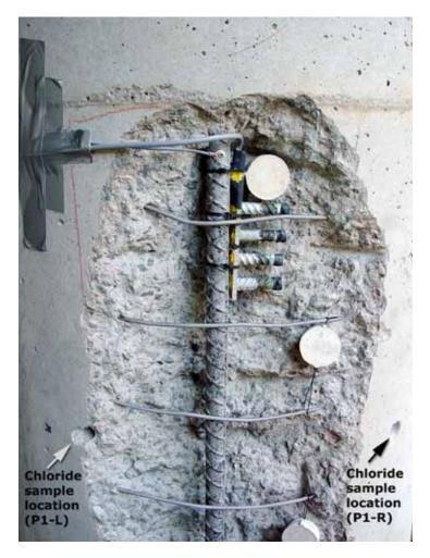
Figure 8. Sacrificial Anode Monitoring Device Placement Before Shotcrete Repair
