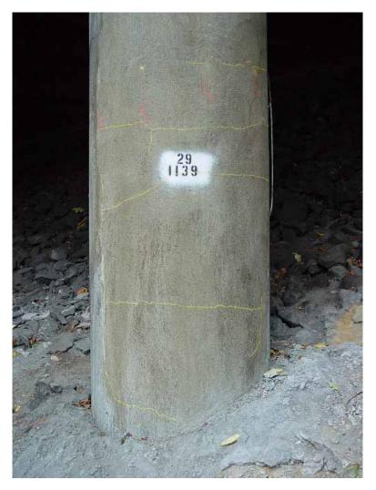
Figure 10. Pattern of Small-width Cracks in a Shotcrete Column Repair
