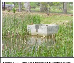
Figure 4.1 - Enhanced Extended Detention Basin (VADCR, 1999).
