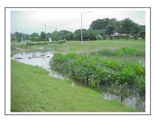
Figure 4.5 - Stormwater Constructed Wetlands (VDCR, 1999)
