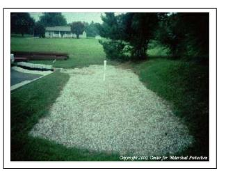
**Figure 4.4 - Infiltration Trench (Center for Watershed Protection)**
