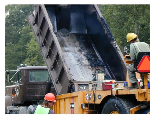
Figure 4. Asphalt Not Sticking in Trucks.
