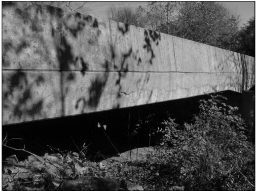
Figure 4. Crack along length of bridge.
