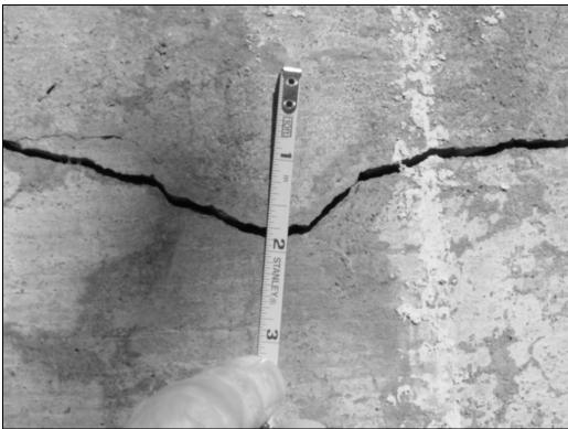
Figure 5. At some locations, crack was 0.25 in at surface.
