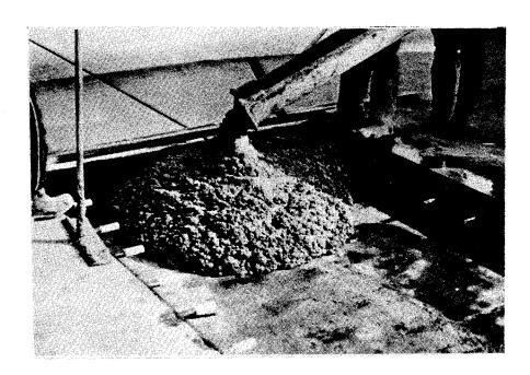
Figure 4. Ready-mix concrete is usually used for large full-depth patches such as large Type C patches or full-depth pavement patches as shown here.
