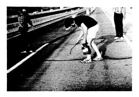
Figure 13. A pressurized spray can be used to apply high molecular weight methacrylate resin to a crack. For best results, a brush should be used to work the resin into the crack.
