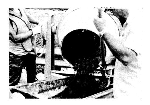
Figure 36. Polyester amide para resin concrete is here discharged into buggy.
