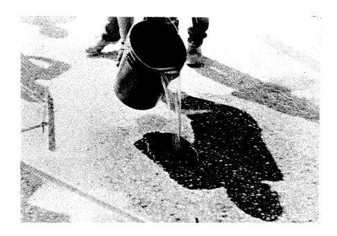
Figure 16. Epoxy should be applied to the deck surface immediately after it is mixed and spread over a premarked area with notched squeeges to insure a uniform application at the specififed application rate. Prior to placing the epoxy overlay, or any type of polymer overlay, the surface should be shotblasted to remove oil, carbonation, laitance, weak surface mortar, and other materials that can interfere with the bonding of the overlay (see Figure 15, pg. 1-8).
