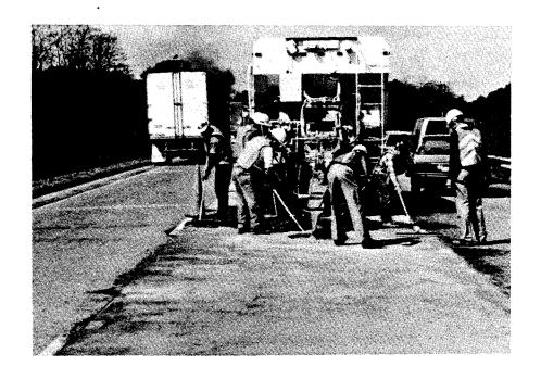
Figure 10. A latex modified slag slurry overlay is applied to a concrete pavement to increase its skid resistance. The surface should be shotblasted prior to placing the slurry (see Figure 15, pg. 1-8).
