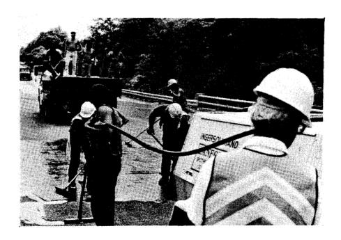
Figure 24. An epoxy wrethane binder that has been blended with positive displacement pumps and mixed with an in-line static mixer is here deposited onto the surface with a wand. Squeeges can be used to spread the resin over the required area and aggregate can be broadcast to excess with shovels from the back of a dump truck.
