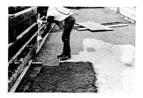
Figure 32. Polyurethane primer can be applied with roller approximately 1 hour prior to placing a premixed polyester amide para resin concrete overlay. The primer must cure prior to the placement of the overlay.
