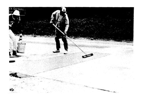
Figure 5. The ready-mix concrete should be consolidated with internal vibrators, struck off, textured with a broom as shown here (other textures may be specified) and covered with burlap and polyethylene or liquid membrane curing material. When the patches must be opened to traffic in much less than 24 hrs, the ready-mix concrete is usually made with Type III cement and accelerating admixtures or special high early strength blended cements.
