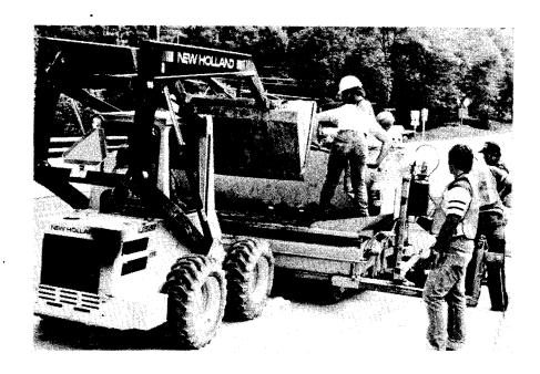
Figure 39. A front-end loader can be used to fill the slip form paver with premixed conductive polyester styrene resin concrete for conductive polymer overlay.
