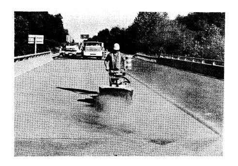
Figure 31. A mechanical sweeper can be used to remove excess aggregate prior to placing a seal coat of methyl methacrylate. The seal coat must cure for at least 30 minutes prior to opening the methyl methacrylate slurry overlay to traffic.
