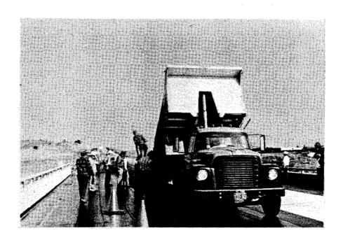
Figure 46. A bituminous concrete overlay should be placed and compacted over the membrane prior to opening the lane to traffic.
