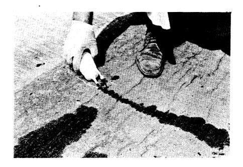
Figure 12. High molecular weight methacrylate can be applied to a crack. For satisfactory filling of the crack, it should be free of debris and wider than 0.1 mm. Also, best results can be obtained by filling cracks when they are open the widest at the surface (temperatures between 55°F and 70°F and between 1:00 a.m. and 10:00 a.m). High molecular weight methacrylate will not cure satisfactorily at temperatures below 55°F.
