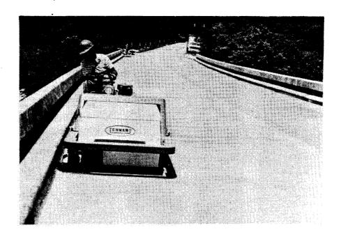
Figure 23. A sweeper-broom type vacuum truck can be used to remove excess aggregate prior to placing the next layer of a multiple-layer polymer overlay.
