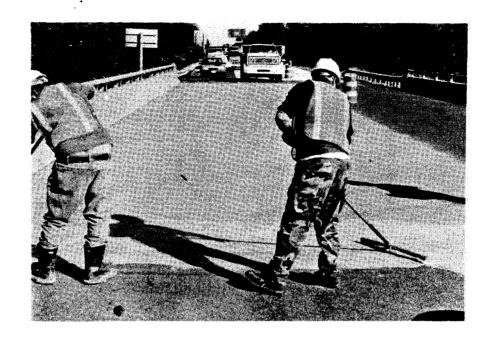
Figure 29. A methyl methacrylate slurry overlay should be struck off with gage rakes set to provide a 3/16 in thick layer of slurry.
