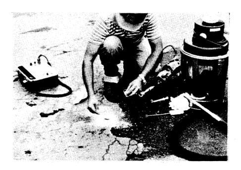
Figure 8. The drill should be returned to the hole, and the sample in the vicinity of the reinforcement should be pulverized. A spoon can be used to collect the sample. A chloride content >2 lb/yd can cause corrosion.
