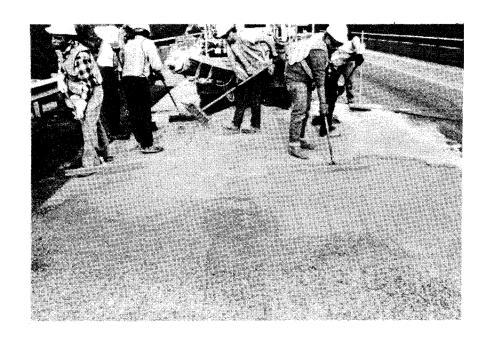
Figure 12. The latex modified slag slurry should be struck off and pulled forward with gage rakes set to provide a 3/16 in to 1/4 in thick slurry. For increased skid resistance slag should be broadcast onto the struck off surface. The slurry should be protected from drying by prompt application of wet burlap and polyethylene when the evaporation rate exceeds 0.05 lb/ft /hr.
