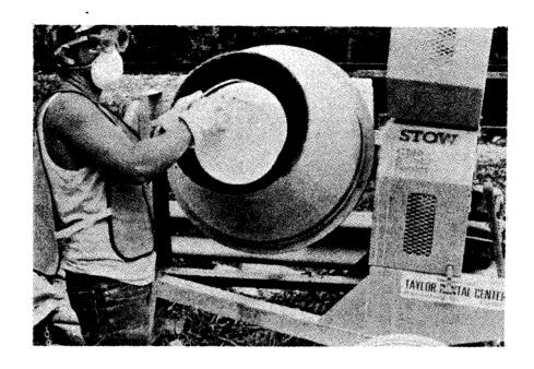
Figure 33. Polyester amide para resin is here added to the concrete mixer.
