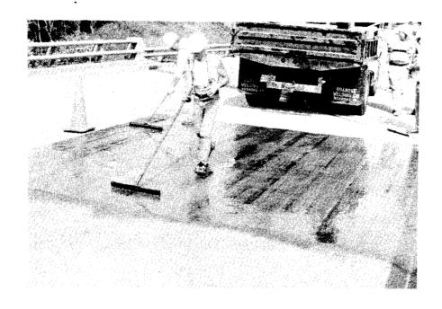
Figure 17. An epoxy urethane mixture is here spread over the deck with notched squeeges. Basalt aggregate is here broadcast to excess from the back of a dump truck.
