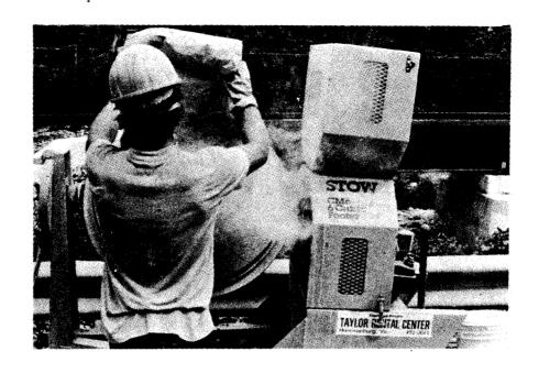
Figure 35. Prepackaged aggregate is here added to concrete mixer.
