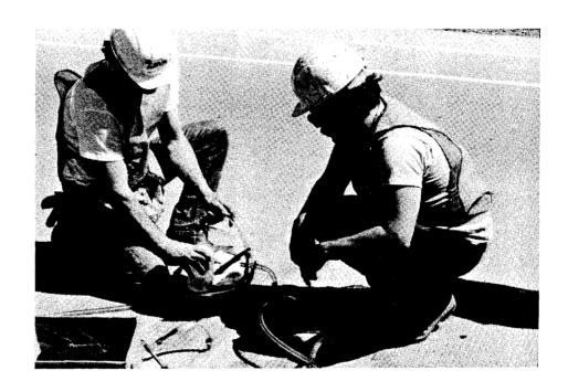
Figure 16. Vacuum injection can be used to fill cracks with a methacrylate resin. Prior to introducing the resin, steel entry ports should be placed on the crack surface, the cracks are covered above and below with a viscous paste-like epoxy, and a vacuum is applied to the cracks through the ports. The requirements for successful filling of a crack cited under Figure 12 (pg 2-7) are also generally applicable to vacuum injection.
