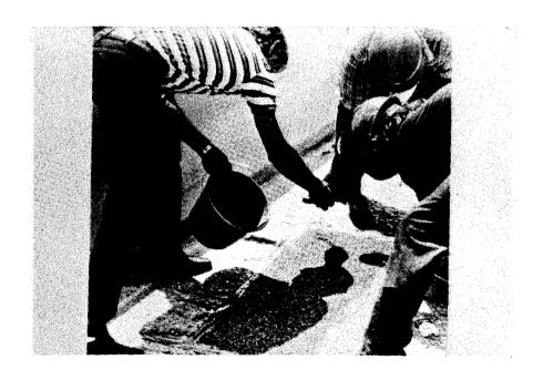
Figure 22. Aggregate should be broadcast onto resin.
