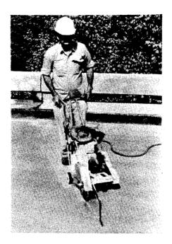
Figure 41. For convenience, polymer concrete overlays may be placed over the joints. The overlay must be sawed over the joint the same day the overlay is placed so that movements of the adjacent spans do not crack and delaminate the overlay.
