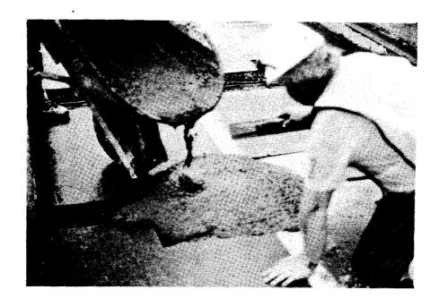
Figure 8. The mixture is usually poured from a wheelbarrow into the cavity. Internal spud vibrators are used to consolidate the concrete.
