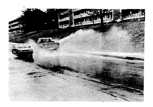
Figure 3. A plugged or improperly located drain (shown above) does not provide for proper drainage. Poor drainage allows water and salt to pond on the surface and to saturate the concrete, which causes freeze and thaw damage in the concrete and creates high salt concentrations at the reinforcing steel.
