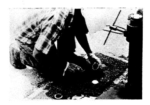
Figure 24. A pipe cap should be bonded to the surface using a rapid-setting adhesive.
