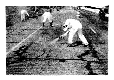
Figure 50. High molecular weight methyacrylate coating can be applied with an airless sprayer. Note that the spray gun operators are wearing impermeable boots, glooves, and coveralls and canister masks.
