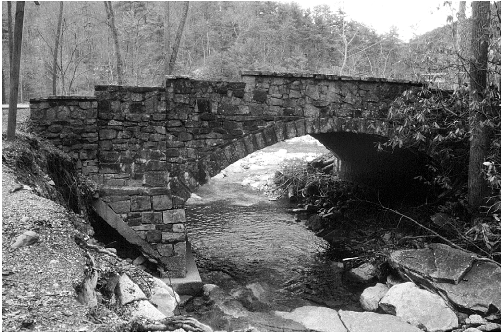
Figure 22. Rigid Frame with Stone Veneer, Built in 1940 as Part of the Improvements to Rt. 39 in Goshen Pass (Rockbridge County Structure No. 1012)
