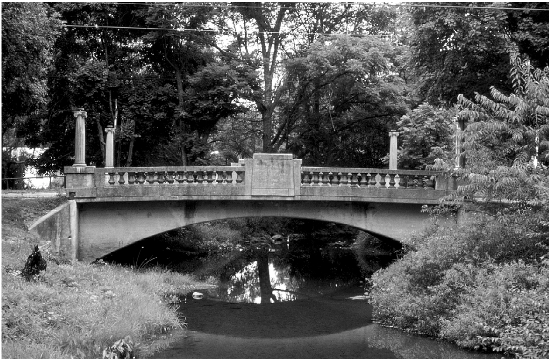
Figure 13. One of Luten's Spandrel Braced Arches, with Decorative Concrete Elements and "Park Rail," Built in 1929 (Bland County Structure No. 1021)
