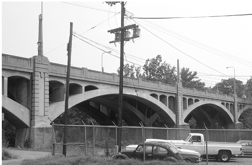
Figure 14. Open Spandrel Rib Arch with Art Deco Design Motifs, Built in 1926 (City of Roanoke Structure No. 1826)
