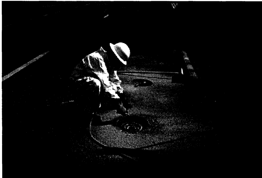
FIGURE 4. POTHOLE BEING CLEANED WITH COMPRESSED AIR
