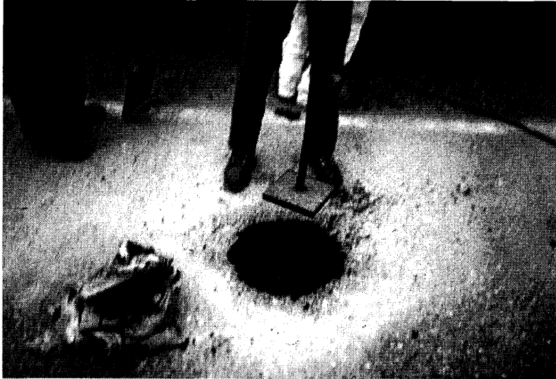
FIGURE 5. PATCHES BEING HAND TAMPED
