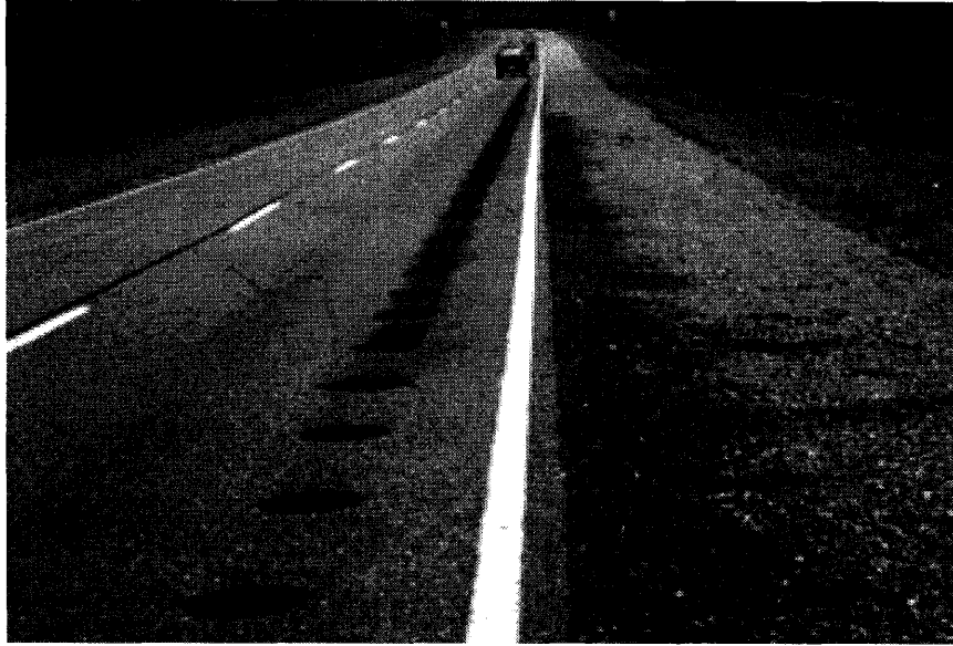
FIGURE 3. MANMADE POTHOLES IN RIGHT WHEEL TRACK
