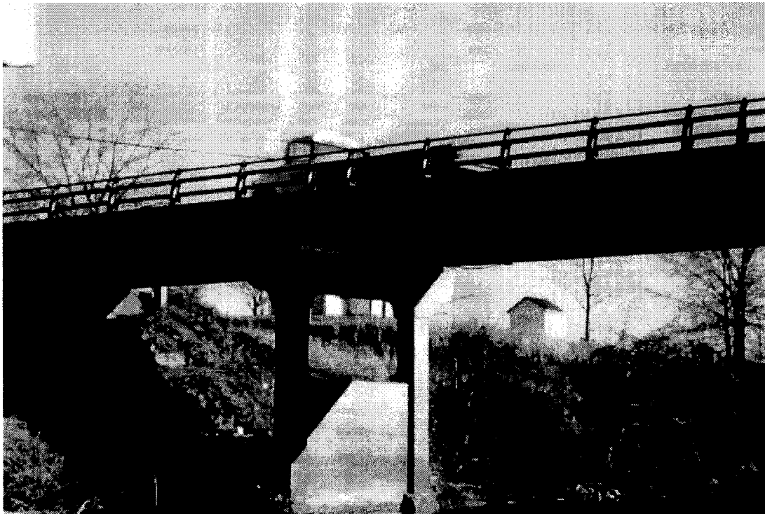
Figure 18. Rte. 29 north-bound bridge over the Robinson River in Madison County, VA.
