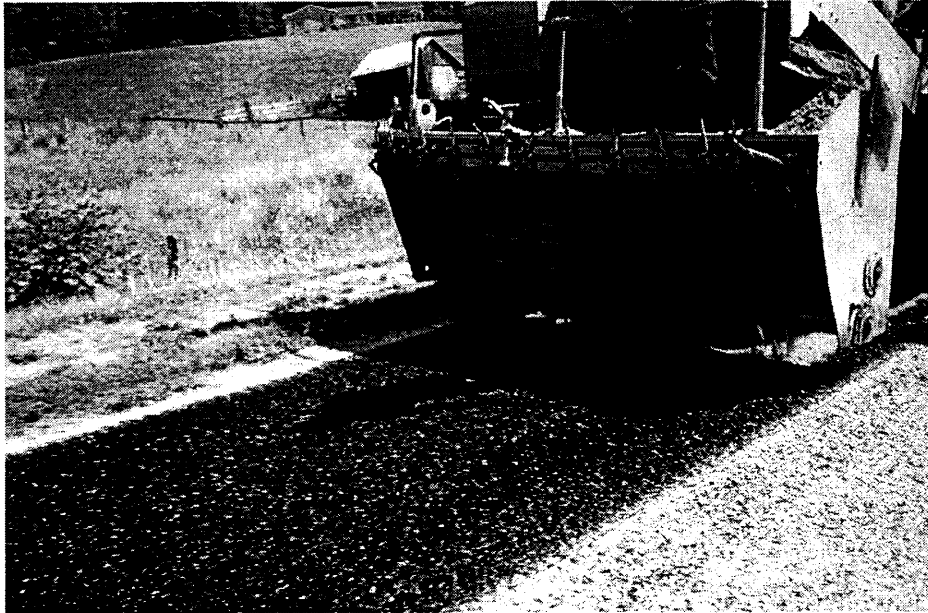
Figure 6. Wet blot material being placed.
