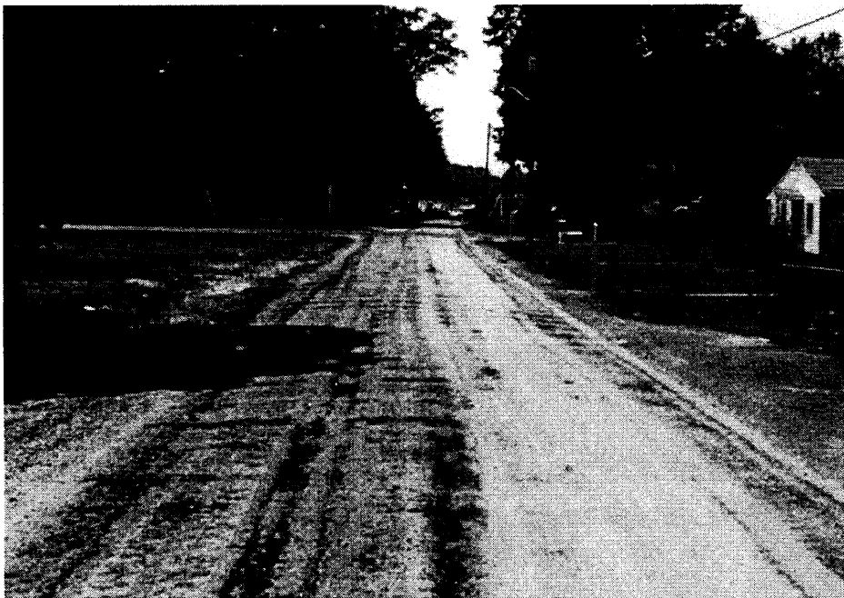
Figure 7. Wet blot material after placement.
