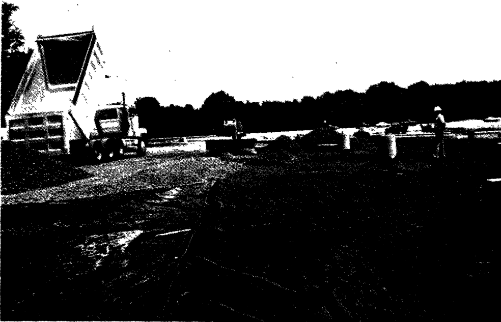
Figure 7. Placement of stone on geotextile.
