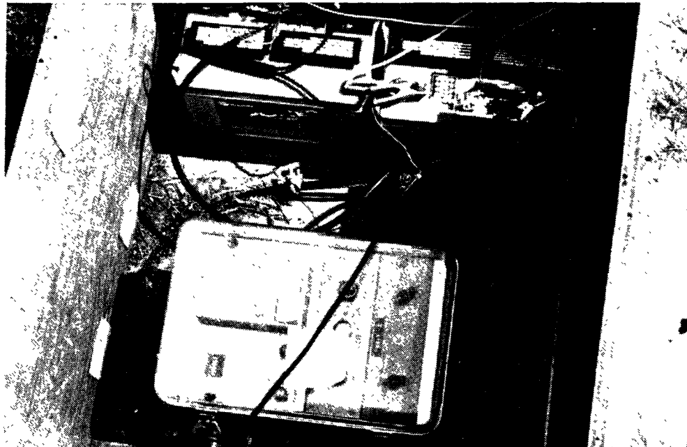
Figure 11. Flow meter with batteries.
