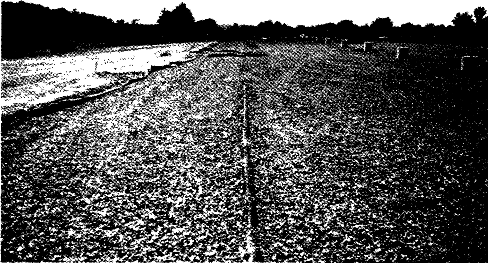
Figure 6. Pipe wrapped in geotextile in No. 57 aggregate base layer.
