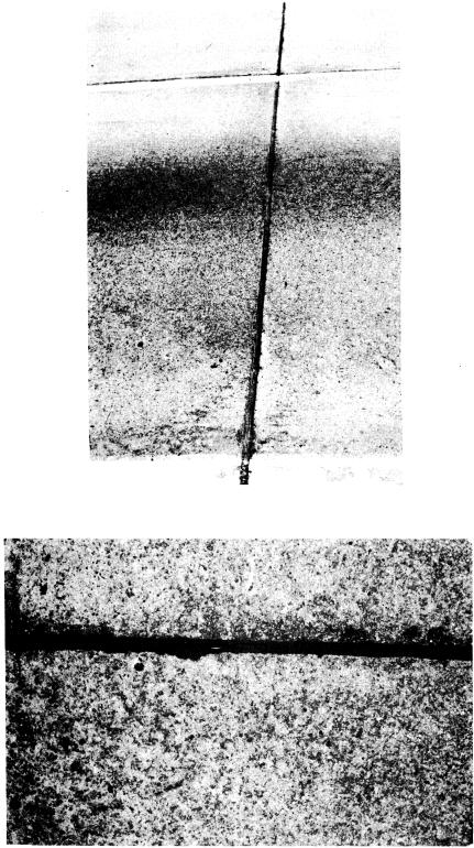
Figure 6. Examples of good (upper picture) and poor performance of polysulfide joint sealants on I-95, Emporia.
