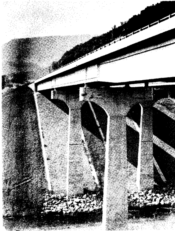
Figure 73. Rte 77 bridge over Laurel Creek in mountainous Bland County.
