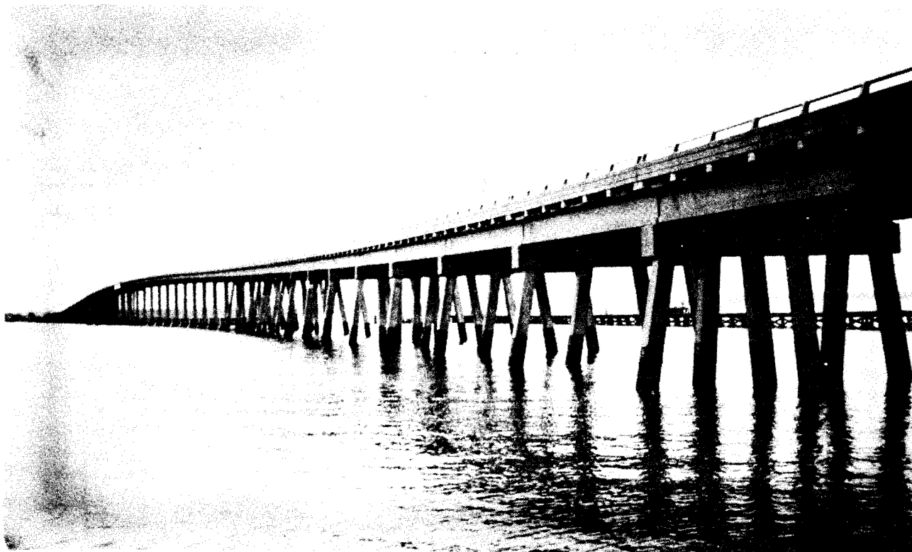
Figure 39. View of bridge from the south bank.
