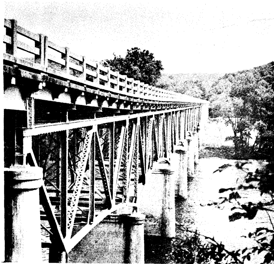
Figure 3. The John H. Cocke Memorial Bridge over James River, showing the large steel trusses.
