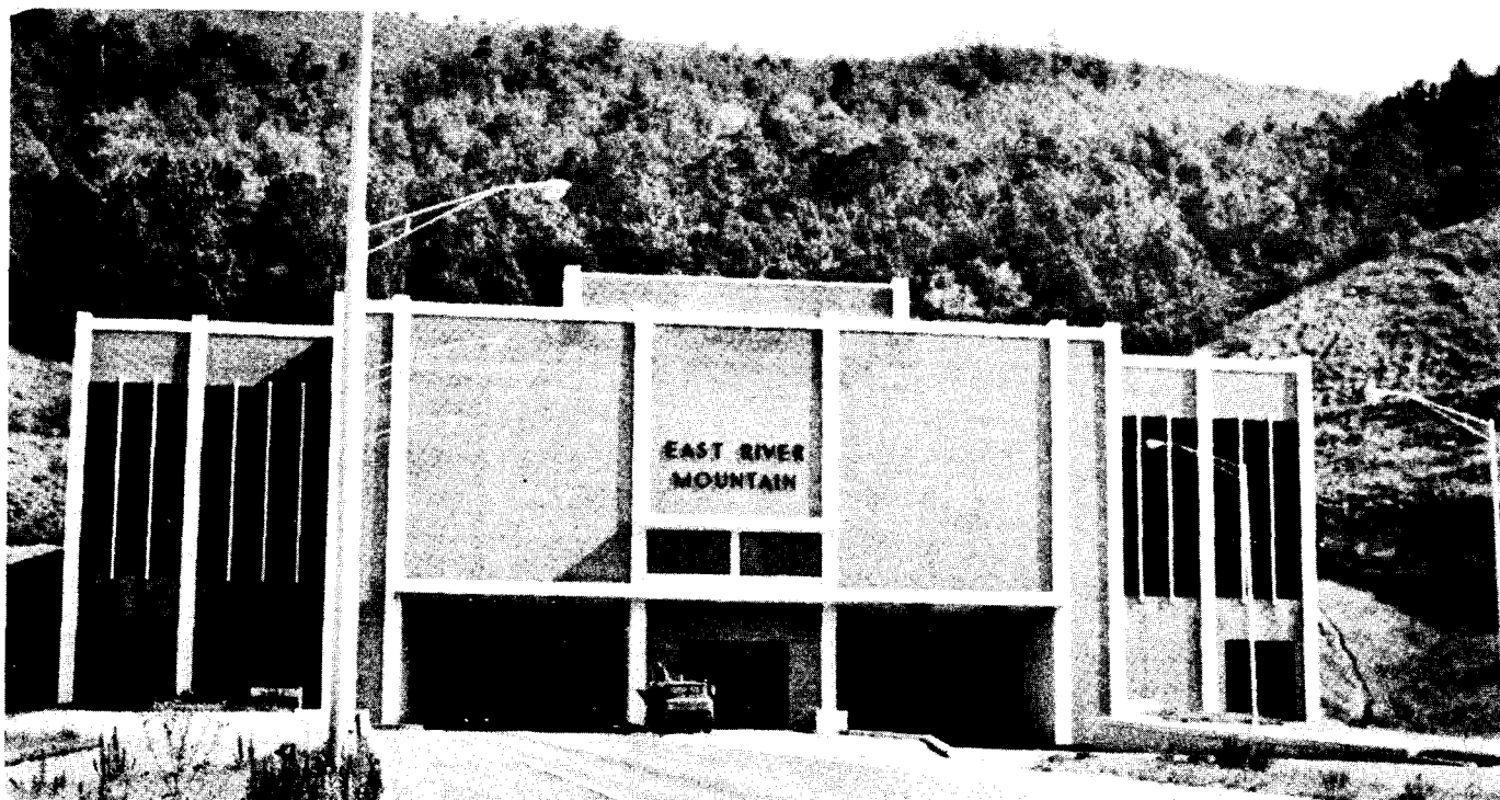
Figure 79. South portal of the East River Mountain Tunnel.
