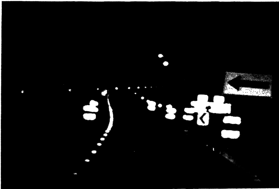
Figure 18. Raised pavement markers and night/wet conditions at Leon.
