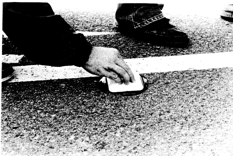
Figure 4. Placement of raised markers on adhesive.
