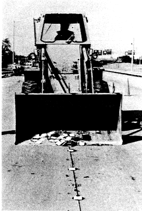
Figure 5. Removal of raised markers.
