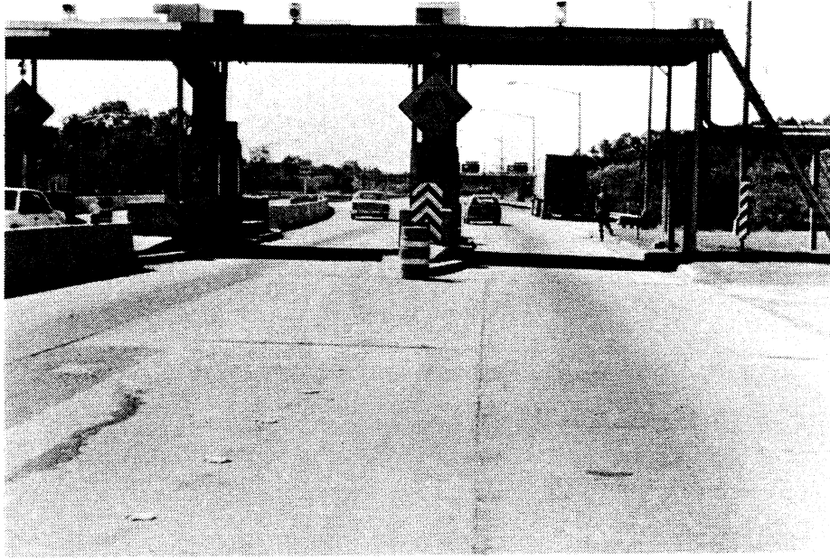
Figure 7. Marker placement on the approach to the toll booths.
