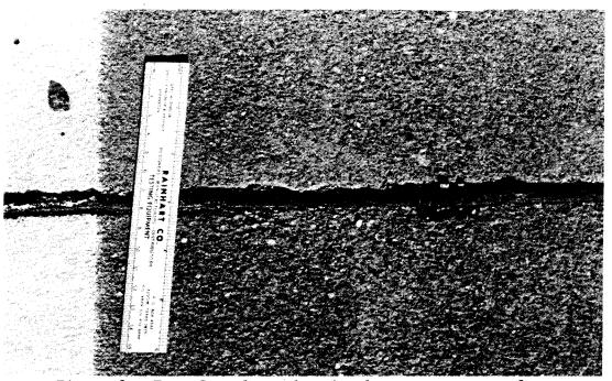
Figure 8. Type C sealant that is above pavement surface.
