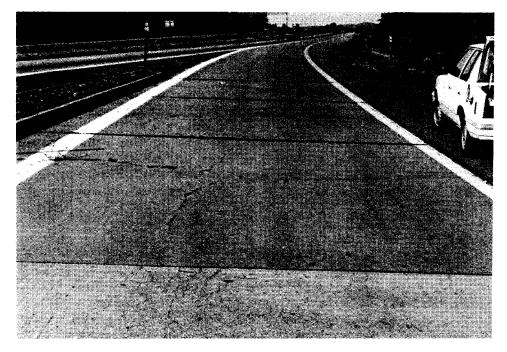
Figure 17. Severely cracked slab adjacent to expansion joints.
