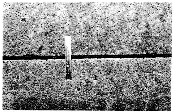
Figure 6. Type A sealant - twisted.
