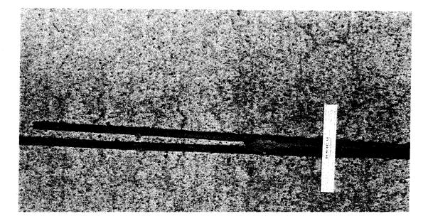
Figure 7. Incorrectly sawn joint.
