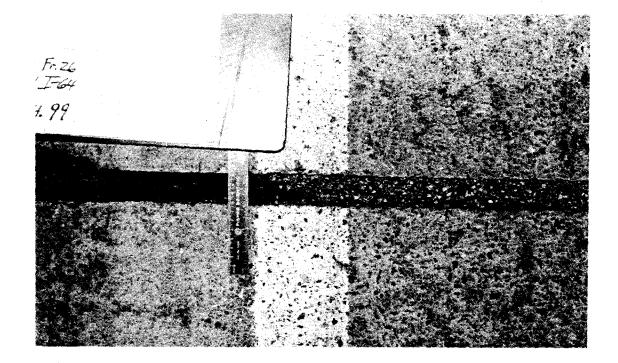
Figure 9. Type A sealant missing at Rt. 631 interchange.
