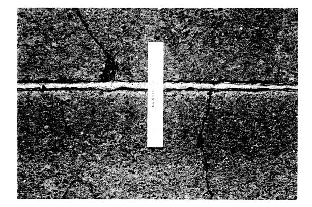
Figure 20. Mildly cracked slabs.
