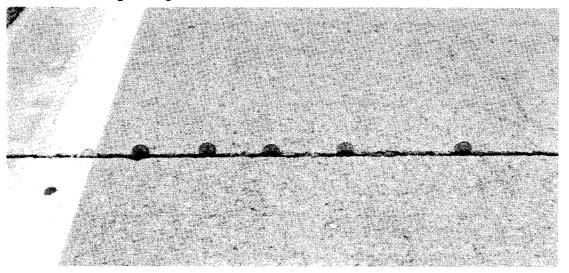
Figure 4. Type A sealant with depths of 0.45 to 0.55 inches.
