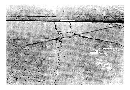
Figure 16. Severely cracked slab at open end of ramp.
