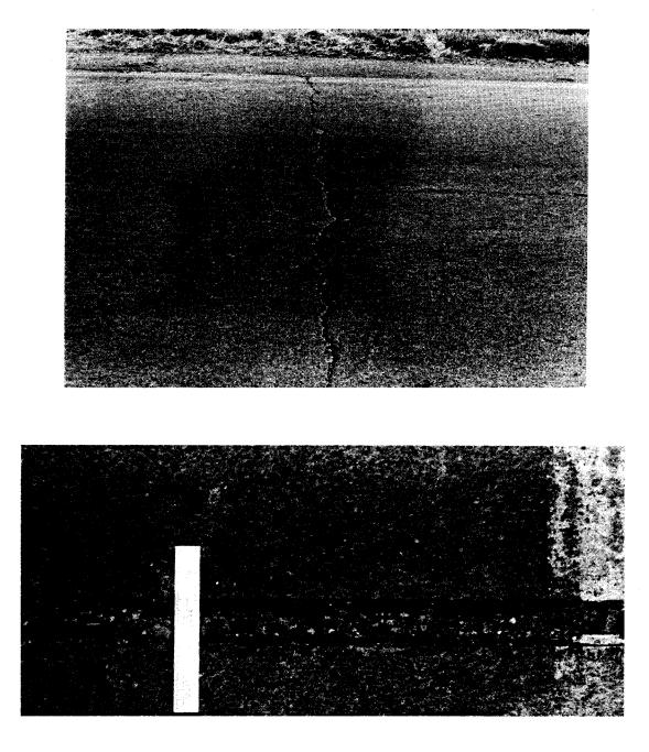
Figure 19. A - Cracking of 1st slab WBL on 250 E. B - 1st Joint - 1/34 inches wide.
