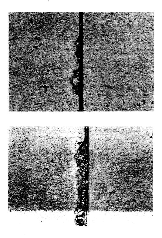
Figure 15. Large spalls.
