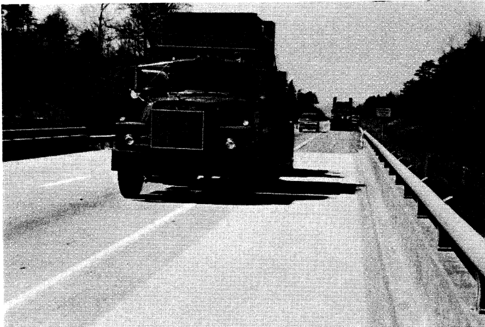
Figure C-2. Shotblast equipment cleans 7-ft-wide path (Rivanna River).
