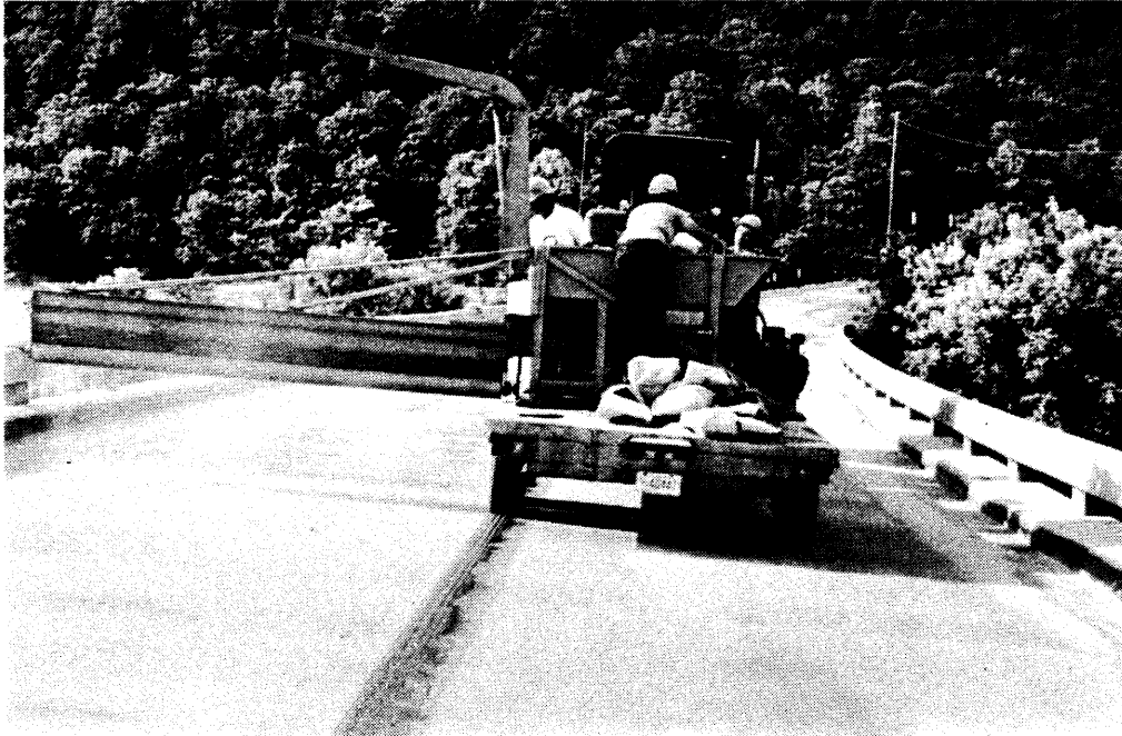
Figure E-2. Application of aggregate with wing spreader (Swan Creek).
