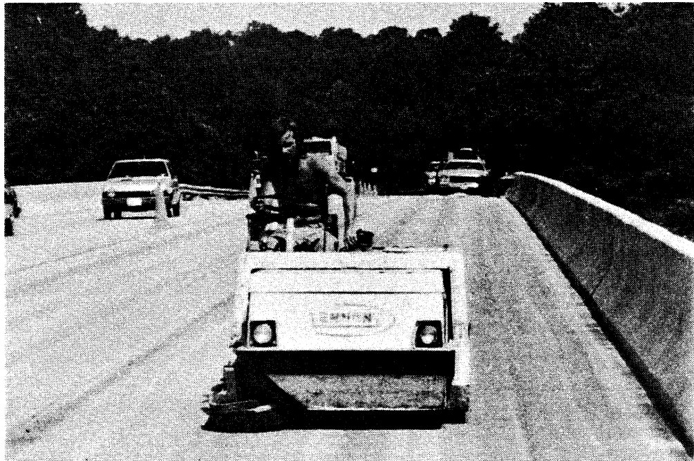
Figure F-1. Sweeper-broom type vacuum truck removes excess aggregate (Williamsburg).
