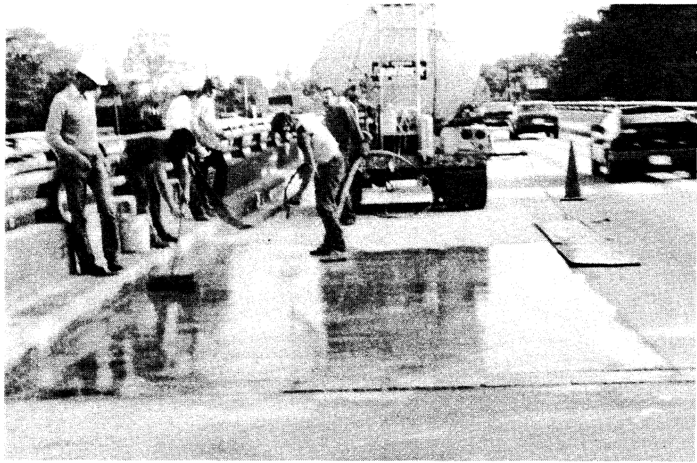
Figure D-1. Spray gun application of resin (Rte. 123 over I-95).
