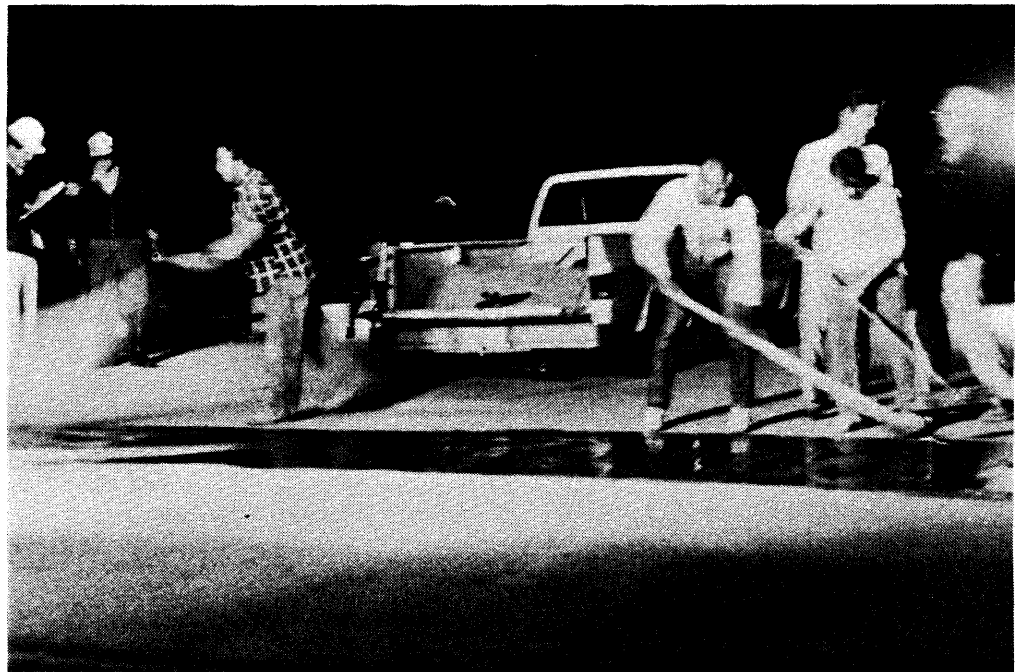
Figure D-2. Hand application of resin and aggregate (frontage road over Rte. 50)
