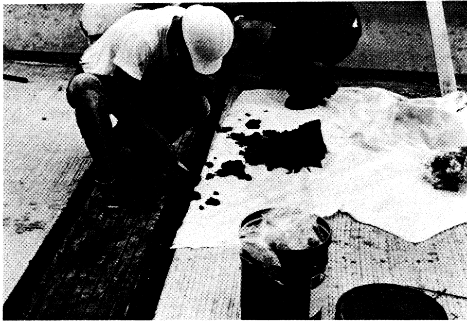
Figure 7. Placing asphaltic material in small troughs on each side of the elastomer.
