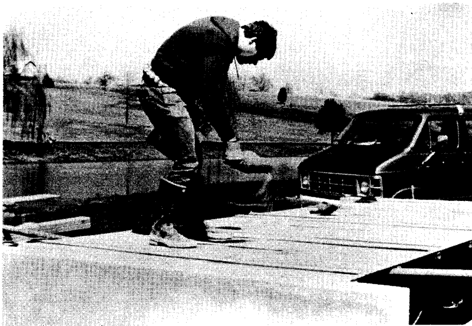
- Figure 6. Sand aggregate applied to polyester resin to form polymer concrete wearing course.
