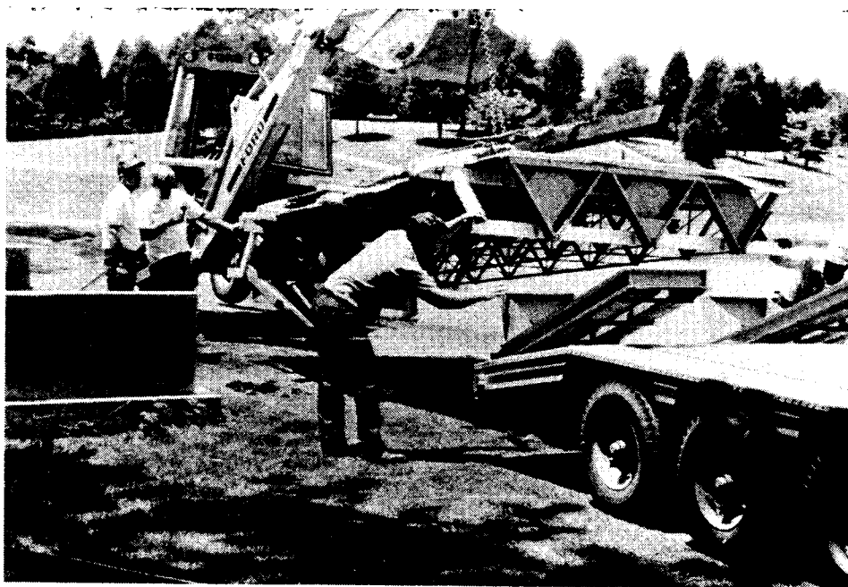
Figure 23. Positioning lowboy trailer beneath suspended superstructure.
