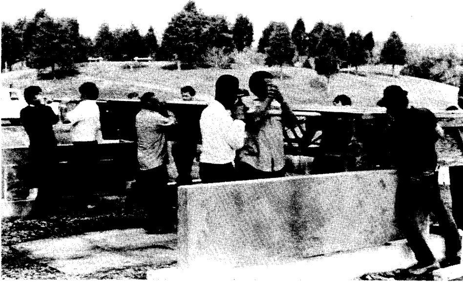
Figure 4. Lifting superstructure onto the precast concrete seats.
