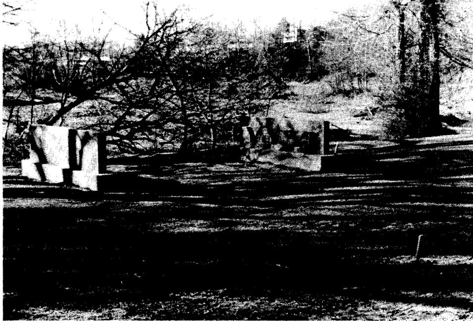
Figure 2. Concrete abutments and precast concrete seats prior to installation of superstructure.
