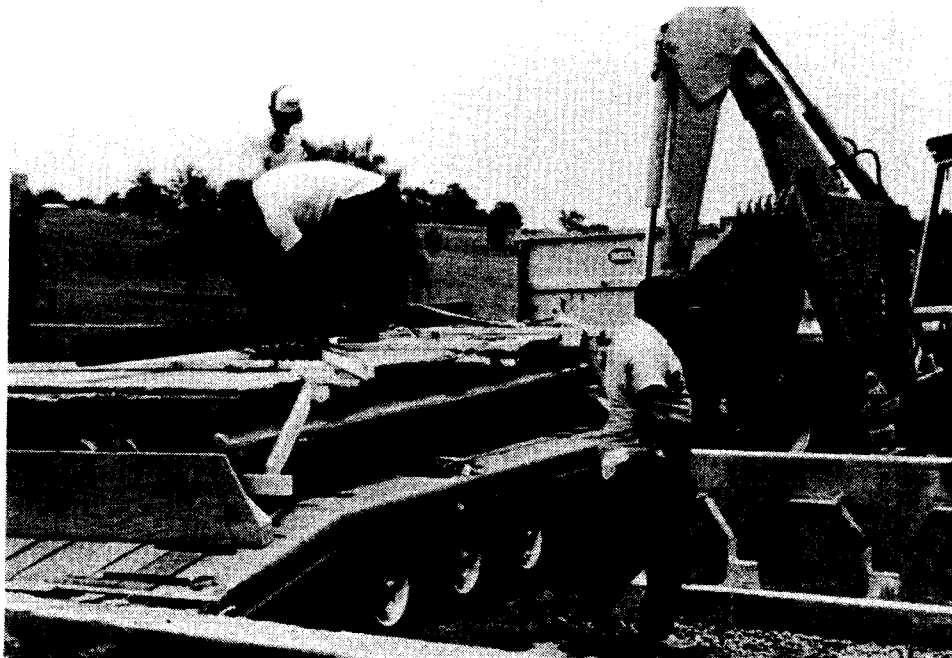
Figure 24. Bridge in place on trailer with temporary wooden supports under the end stiffeners.
