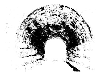
Figure 21. The original stone masonry arch portion of this N & W Railroad underpass in Montgomery County is visible between two concrete barrels which were added later to widen the bridge.
