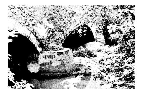
Figure 4. Two-span stone arch bridge on the nineteenth century Snicker's Gap Turnpike corresponds to the construction types in Figures 2 and 3, and could have been built by the same mason. This route is further clarified by their description of tollgate locations:
