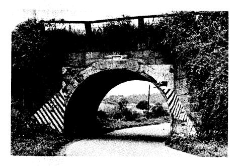
Figure 16. The keystone carving of 1901 on this N & W Railroad underpass dates this arch to an era of very late solid masonry construction.
