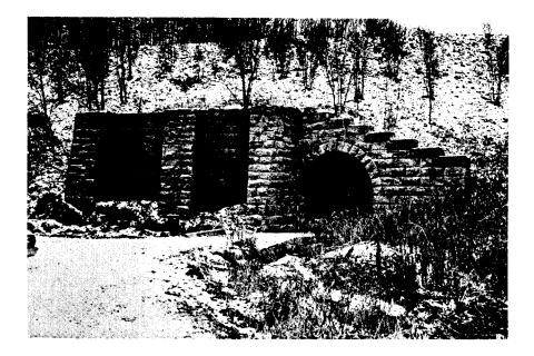
Figure 12. This asymetrical, massively buttressed railroad underpass was built at Honaker by the N & W Railroad between 1887 and 1889 on its Clinch River Extension, which tapped rich coal fields.
