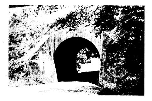
Figure 31. Concrete arch underpass, constructed in Montgomery County, illustrates the regional diversity found in Virginia arch types. This "horseshoe arch" was built only in Montgomery County. Figure 32 shows a multi-span, low arch bridge typical of Shenandoah County design and encountered elsewhere only in 2 bridges in Montgomery County.
