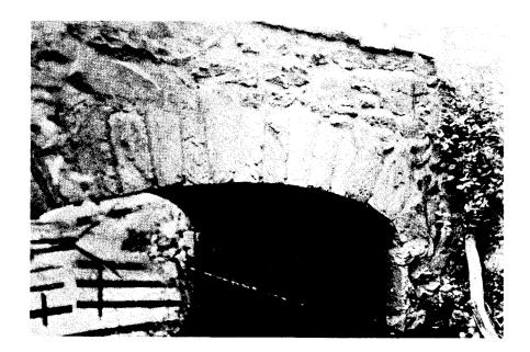
Figure 6. Single-span stone masonry bridge, also located in Loudoun County, is similar to that in Figure 5. These may be small-span nineteenth century turnpike bridges, termed "large stone culverts" in the Public Works records. To the west, in the Staunton District, are 2 small-span masonry arches like those of Figures 5 and 6. They may be bridges which carried the Huntersville-Warm Springs Turnpike, or they may date to a later period.
