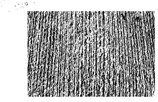
Figure 7. Scoring on deck of Route 220 NBL bridge over Route 419.
