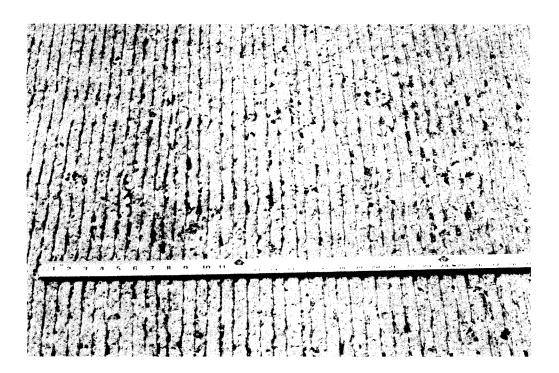
Figure 2 View of striations impressed by the Flexi-Glide tine. Note the harsh texture between the striations.
