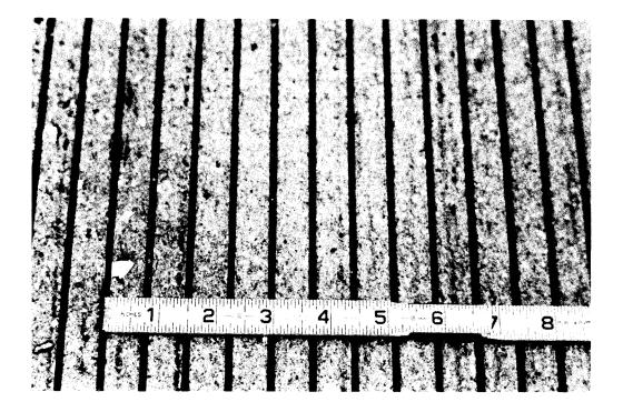
Figure 12 Grooves sawcut into hardened concrete deck.
