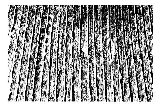
Figure 6. Deck striated with leaf rake.
