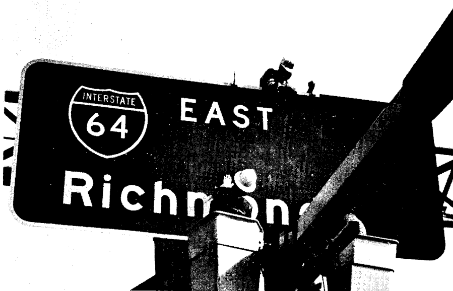
Figure 3. Riveting overlay panel to in-place sign.
