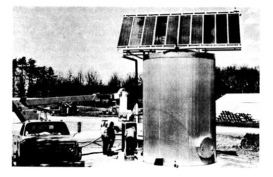
Figure 2. View of completed solar heated asphalt storage tank.
