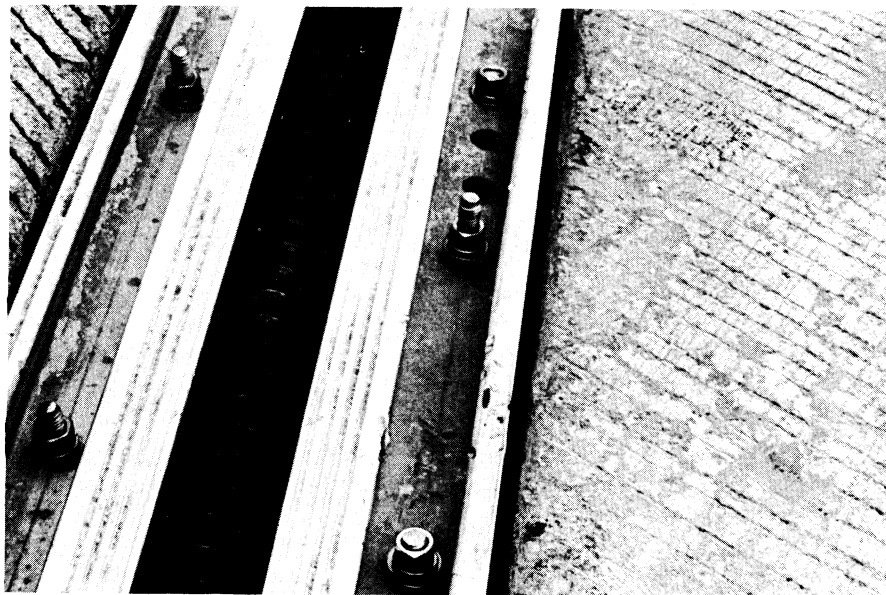
Figure 4. View showing irregular anchor bolt spacing required when reinforcing steel in the concrete prevented hole drilling at the planned location. Note also, at the center of the photograph, the extra washers used to elevate the nut after pullout of some of the anchor bolts occurred during tightening.
