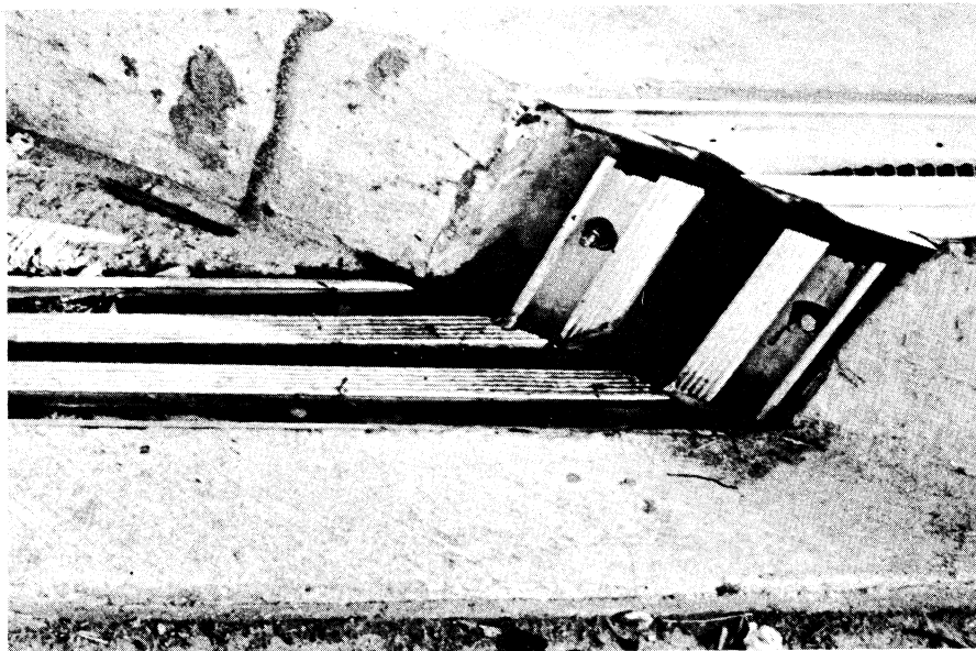
Figure 13. Appearance of the joint at the face of the median strip on the Duke Street bridge.
