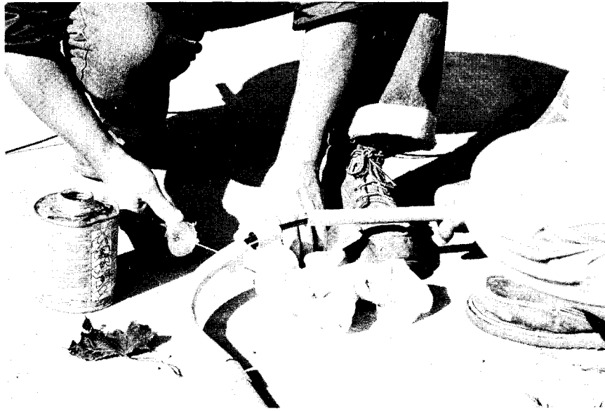
Figure 3. Gluing PVC loop.
