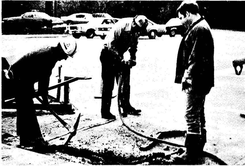
Figure 5. Breaking out the saw cuts for PVC loop.
