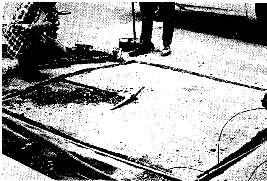
Figure 8. PVC loop in saw cut.
