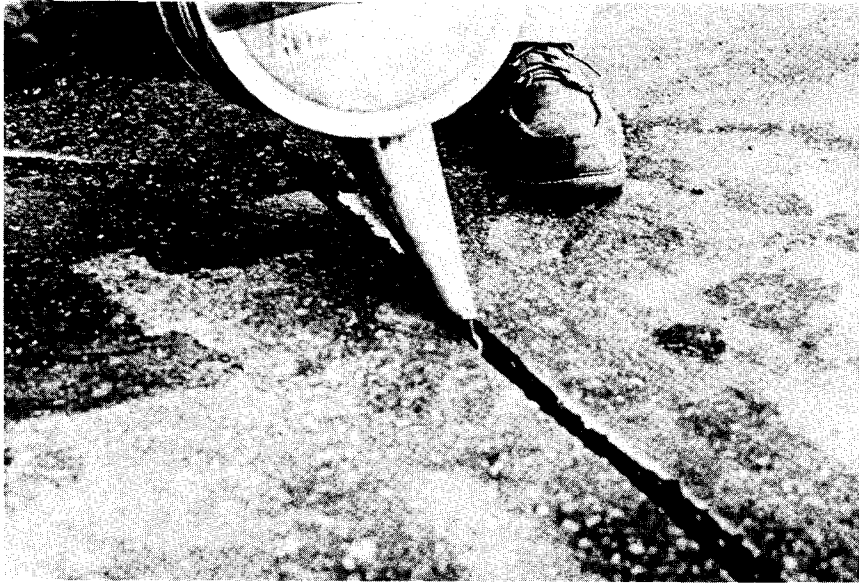
Figure 15. Filling cut for plastic loop with sealant.
