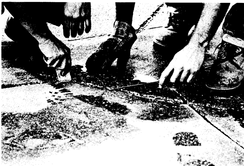
Figure 14. Placing plastic loop in cut.
