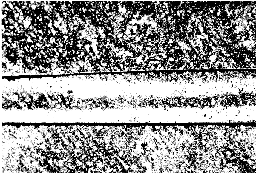
Figure 4. Parallel saw cuts for PVC loop.
