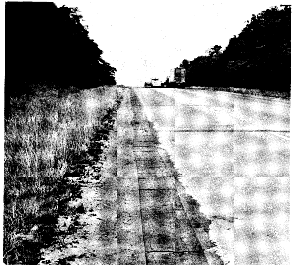
Figure 2. Installing fabric over pavement shoulder joint (left), and finished job.
