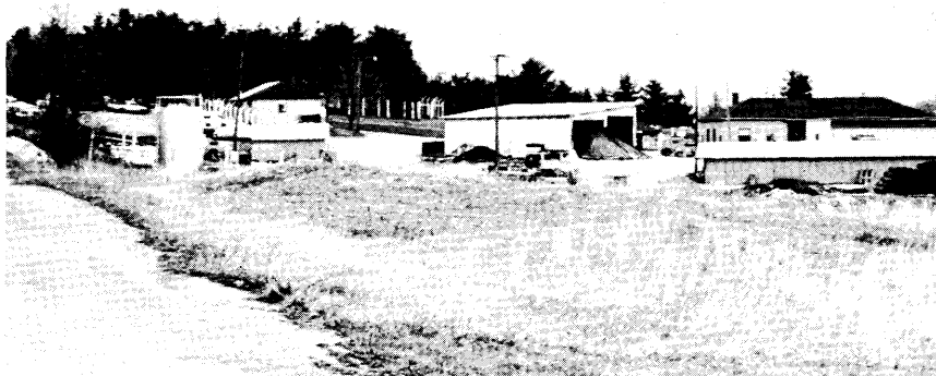
Figure 6. Distant view of Christiansburg residency complex. Anemometer is on pole to left of tower.
