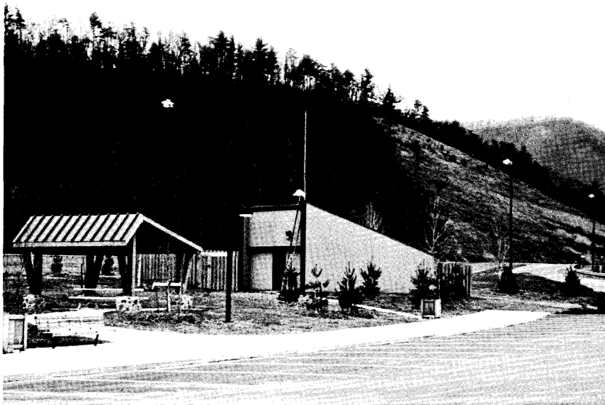
Figure 8. View of pump house, looking south, with Hogback Mountain in background.
