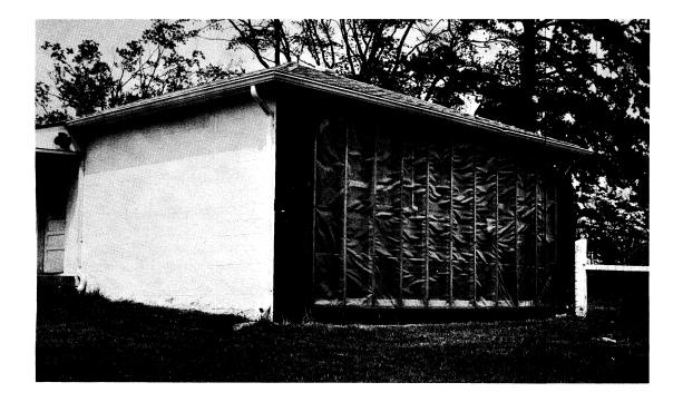
Figure 10. Trombe wall retrofitted on the Yancey Mill area headquarters office.
