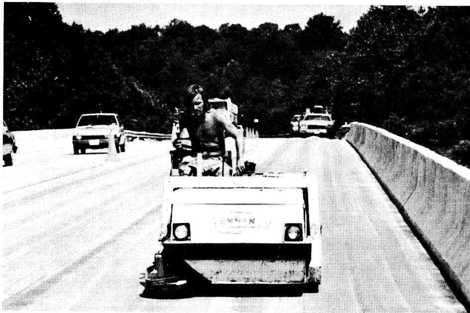
Figure 7. Sweeper-broom type vacuum truck removes excess aggregate.
