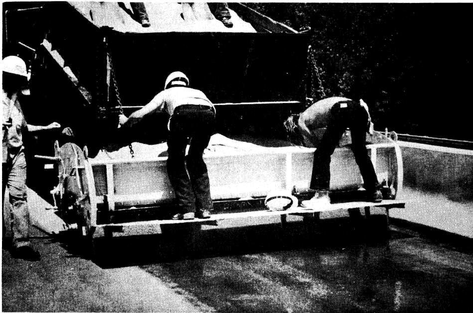
Figure 2. Silica aggregate is broadcast over resin.
