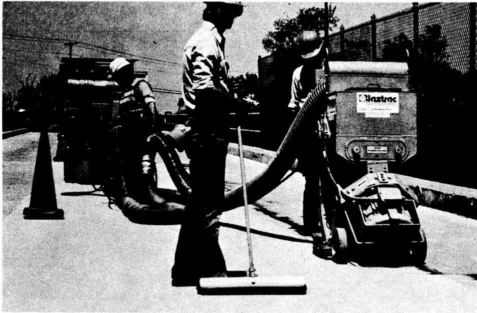
Figure 5. Shotblasting equipment similar to that used on the bridges near Williamsburg.
