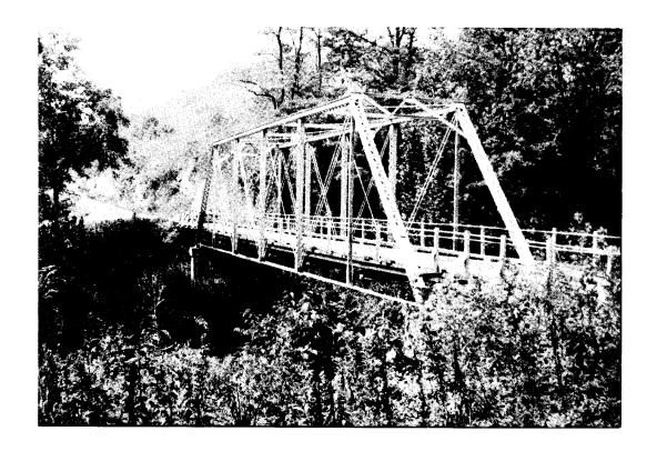
Figure 10. A single-span Pratt through truss built by the Penn Bridge Company of Beaver Falls, Pa.
