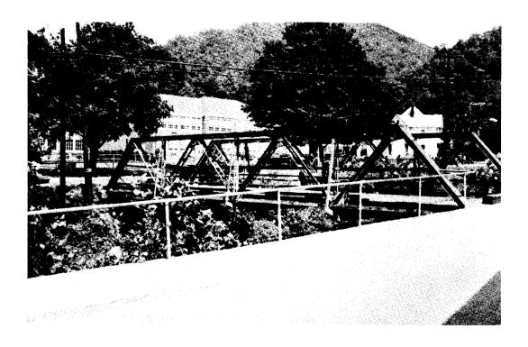
Figure 11. A typical twentieth century pony truss with riveted connections built by HIPCO Steel Bridges in 1925.
