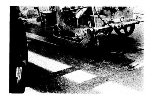
Figure 7. Applying thermoplastic material.
