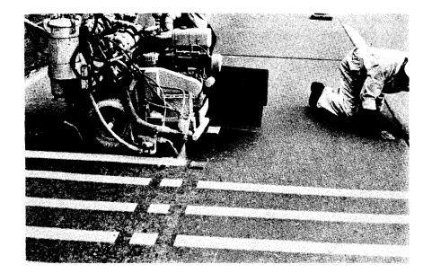
Figure 5. Applying test stripe on pavement and sample plates.
