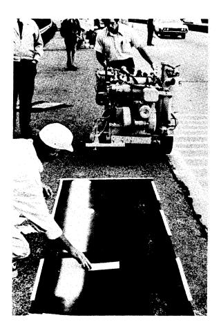
Figure 2. Calibrating for paint thickness.
