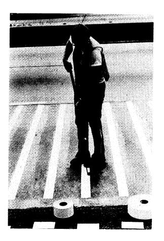
Figure 8. Applying preformed tapes.
