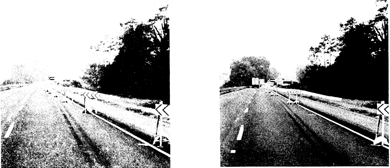
Figure 5. Views of the 40-ft. (12.3 m) and 80-ft. (24.6 m) spacings for the Type I chevron barricade.
