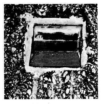
Figure 6. Mono-directional red marker in place.
