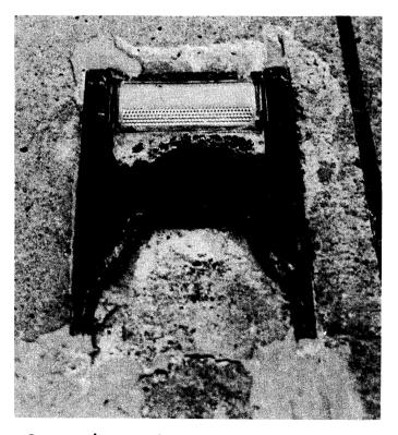
Figure 8. Steel casting and marker on pavement surface.
