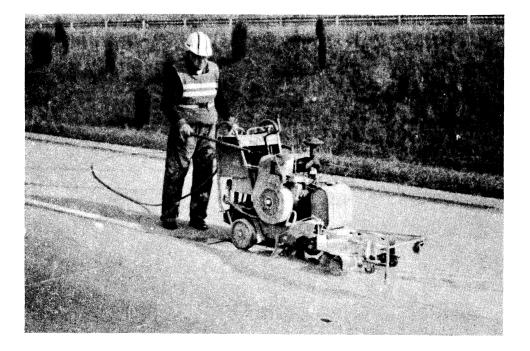
Figure 4. Cutting groove in pavement.
