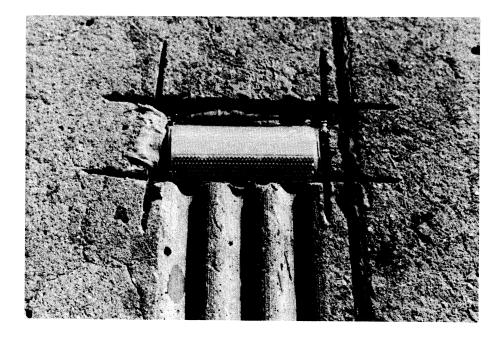
Figure 7. Marker emplaced in concrete pavement.
