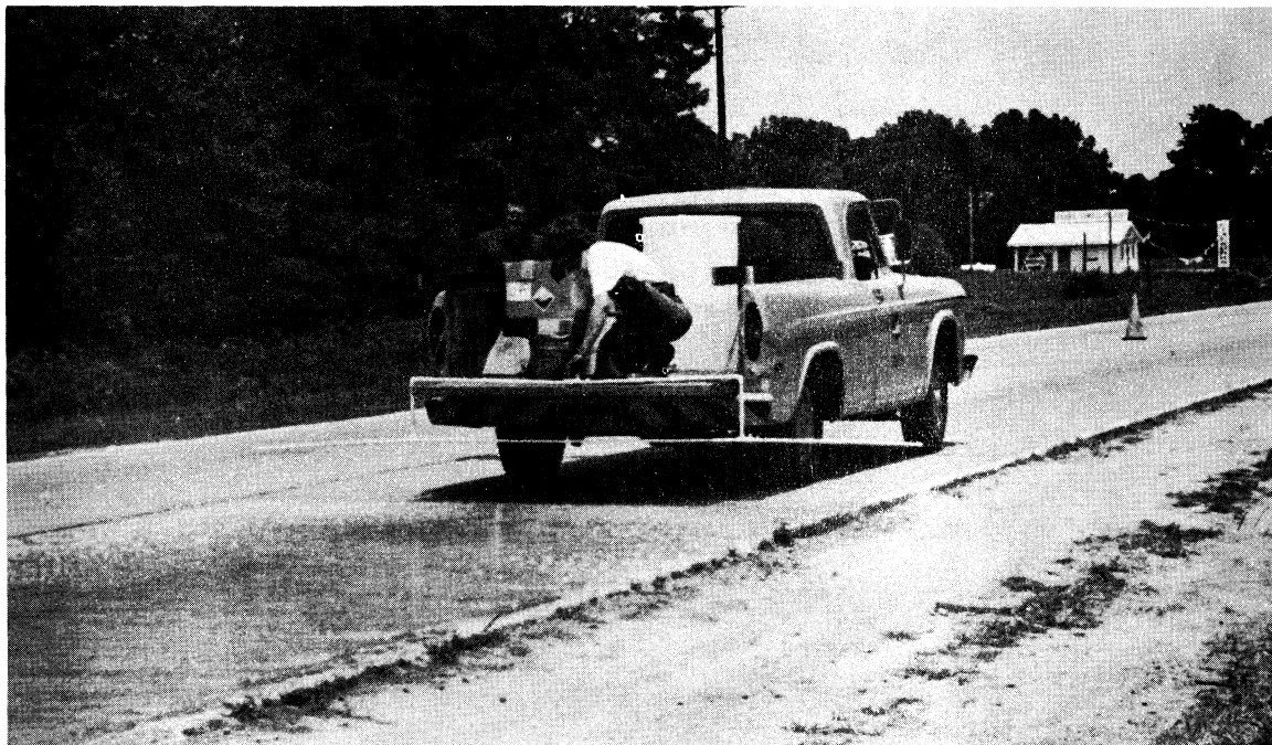
Figure 6. Acid being applied to roadway.
