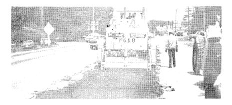
Figure 3. Pettibone pulverizer in use.
