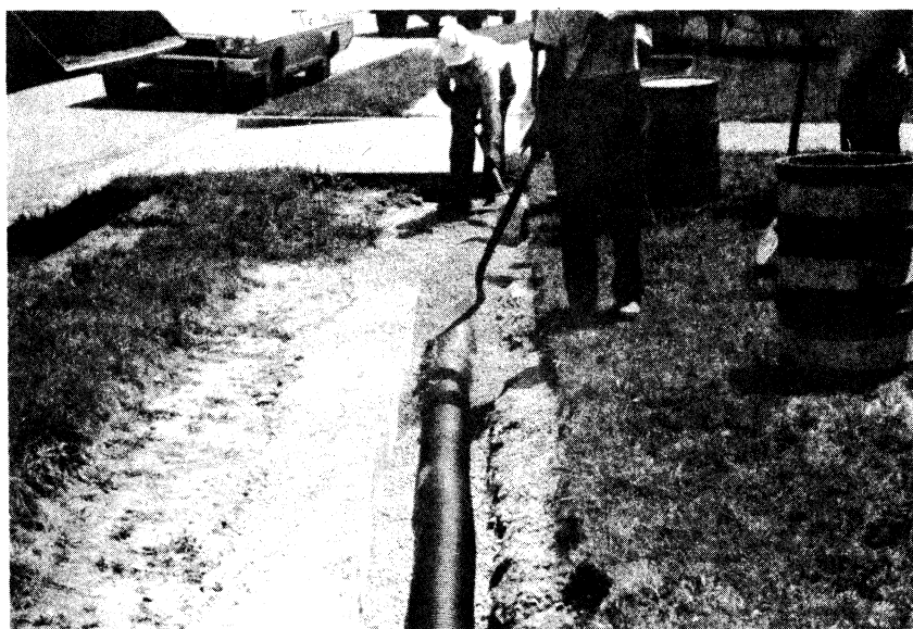
Figure 3. Sidewalk replacement utilizing curtain wall and subsurface drainage.
