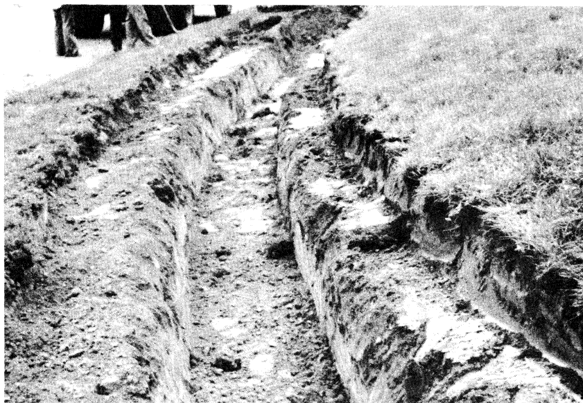
Figure 9. Test site showing erosion channel after shaping.
