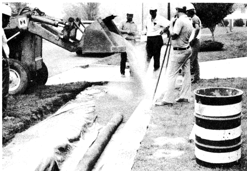
Figure 10. Test site showing installation of polyethylene, pipe, and No. 8 stone.
