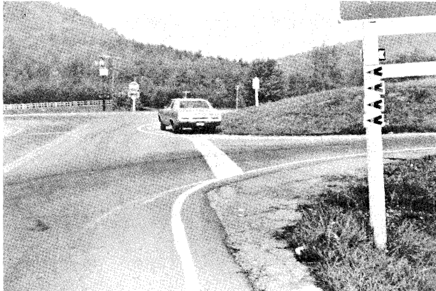
Figure 2. Intersection 43 on I-81 S. Nonvisibility of the pavement arrow marking from the crossroad when placed 22 feet from the stop line.
