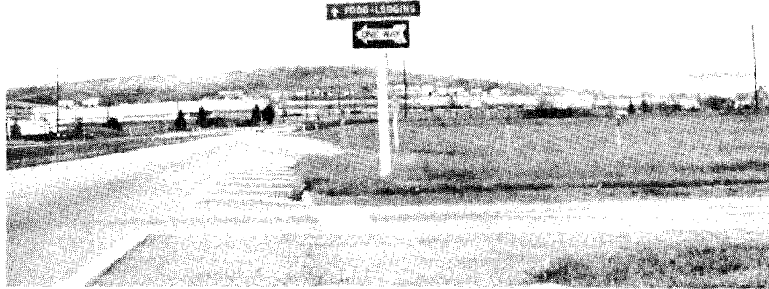
Figure 1. Intersection 59 on I-81. Visibility of pavement arrow marking when placed near the stop line.
