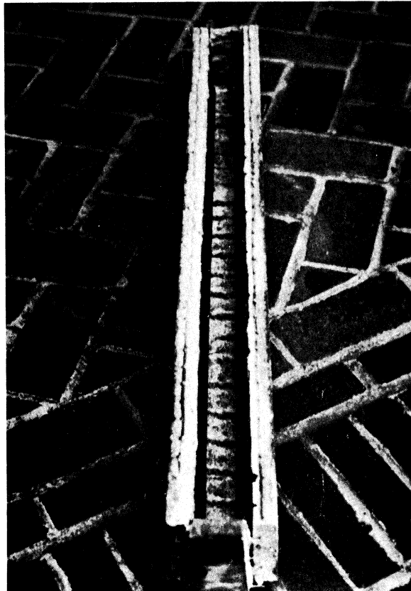
Figure 4. Shell with reinforcing steel.
