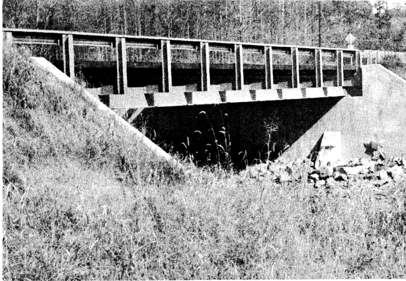
Figure 1. Fairfax County bridge.
