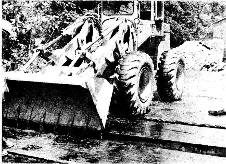
Figure 5. Front-end loader used to pull panels together on Patrick County bridge.
