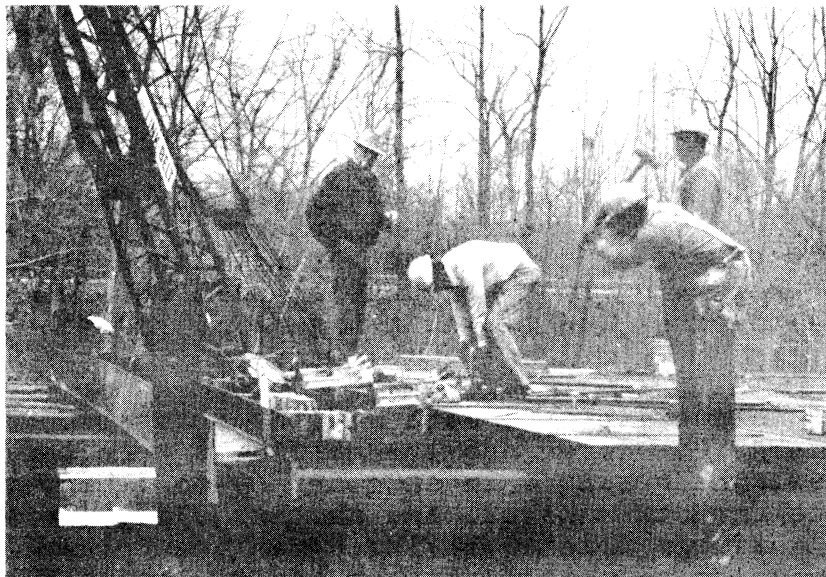
Figure 2. Panels are jacked together on Fairfax County bridge.
