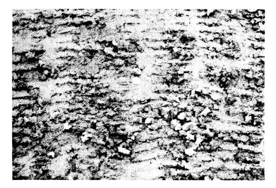
Figure 14. Raked surface of stage one concrete with quarter dollar shown for size.
