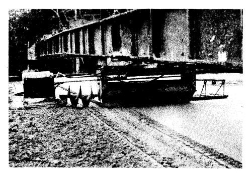
Figure 13. Transverse screed used in placement of overlay concrete.
