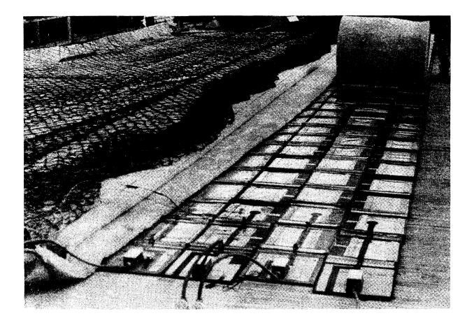
Figure 20. Heating blankets on deck with insulation and netting.
