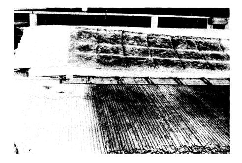
Figure 22. Transition on deck between unheated concrete (left) and darkened, heated concrete (right).
