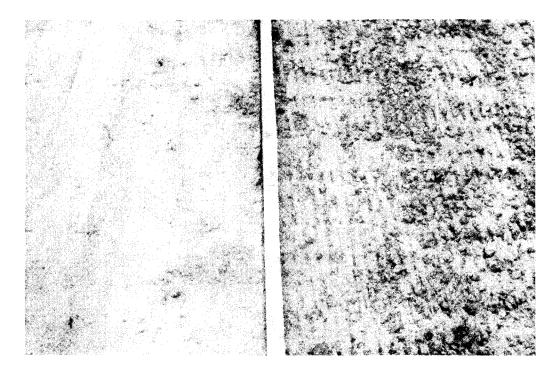
Figure 15. Stage one concretes at expansion joint showing screeded finish (left) and raked finish (right).
