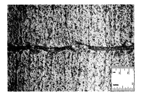
Figure 7. Transversely tined texture, grooves spaced on 76 mm (3 in.) centers. Site 2.
