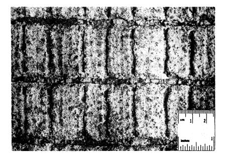
Figure 15. Tined texture with grooves spaced on 19 mm (3/4 in.) centers longitudinally and 38 mm  $(1 \ 1/2 \text{ in.})$  centers transversely. Site 10.
