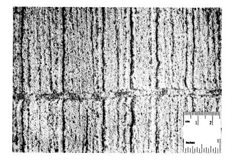
Figure 13. Tined texture with grooves spaced on 19 mm (3/4 in.) centers longitudinally and 76 mm (3 in.) centers transversely. Site 8.
