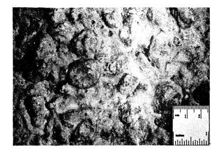
Figure 9. Sprinkled aggregate texture with 19 mm (3/4 in.) maximum size aggregate. Site 4.
