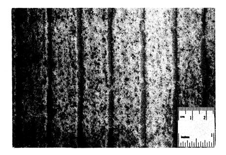
Figure 6. Longitudinally tined texture, grooves spaced on 19 mm (3/4 in.) centers. Site 1.
