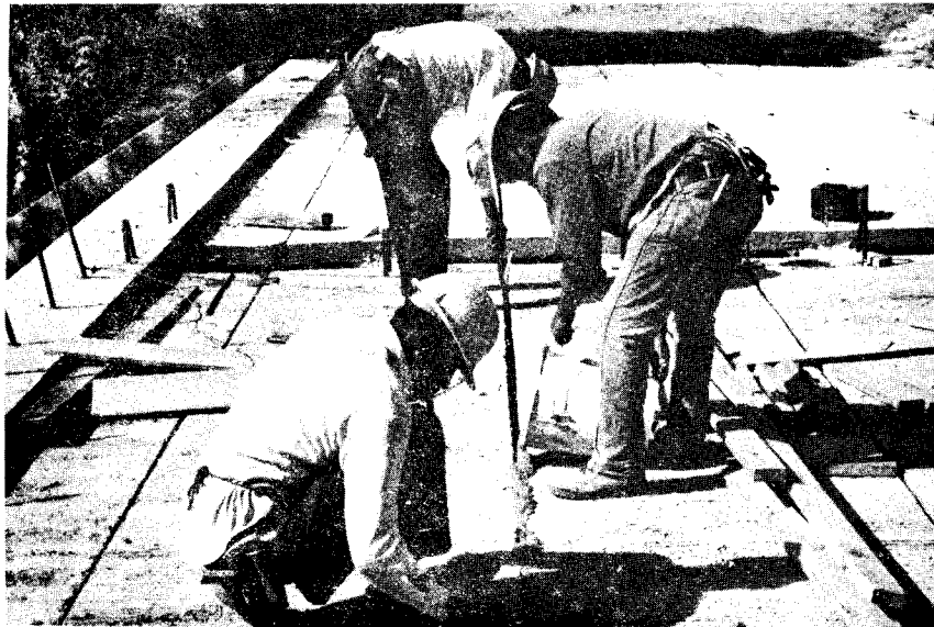
Figure 4. Nonshrinking cement paste placed between adjacent tee beams.
