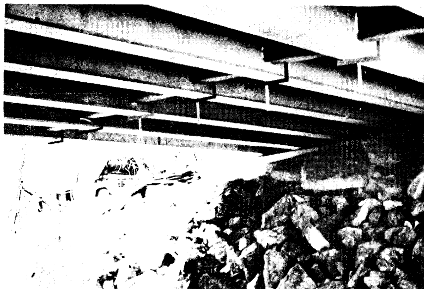
Figure 24. Scales attached at midspan for measuring beam deflections as the overlay was placed.
