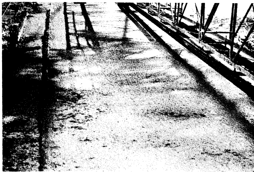
Figure 48. Variable consistency concrete pulls in lower part of figure and flows in upper part.
