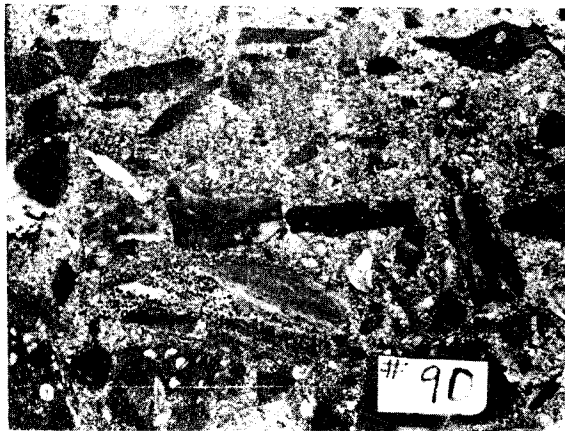
Figure 46. Core from span B of B602 shows that much of the cement mortar and air has been lost.
