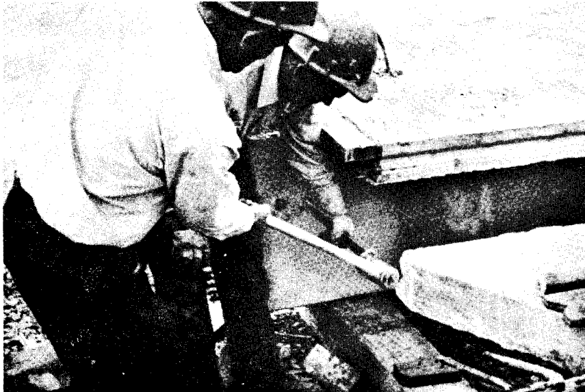
Figure 11. Inserts that provide voids for the diaphragm steel are removed.
