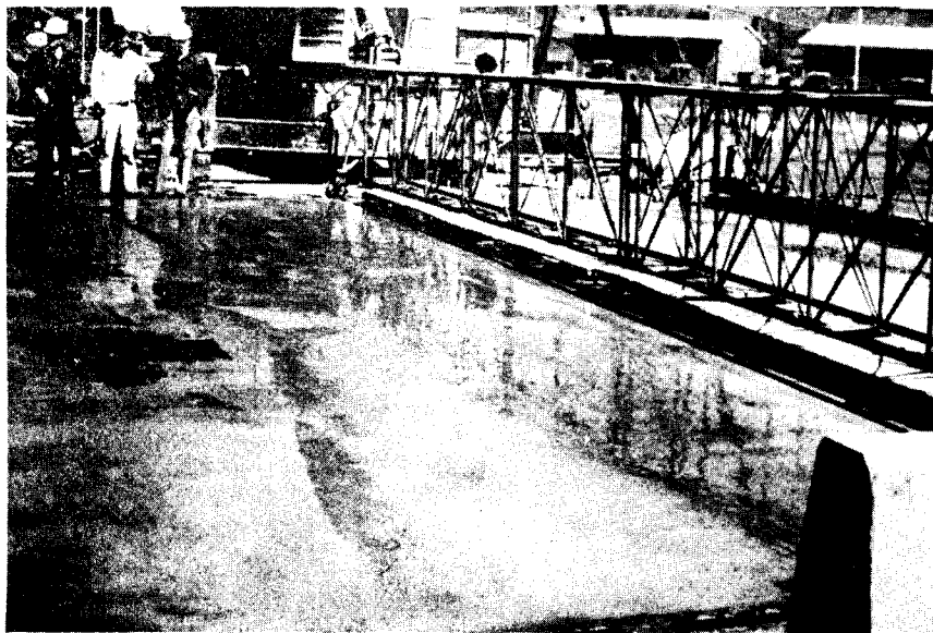
Figure 47. Excess bleed water covers most of span C of B603 as screeding and finishing operations are completed.
