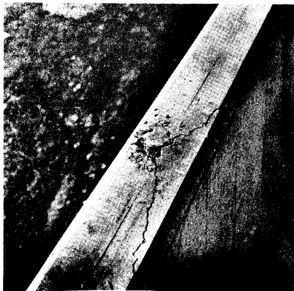
Figure 32. Structural cracking and spalling of precast parapets in vicinity of mortar-filled void.
