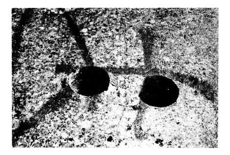
Figure 5. Core holes showing incipient spall.
