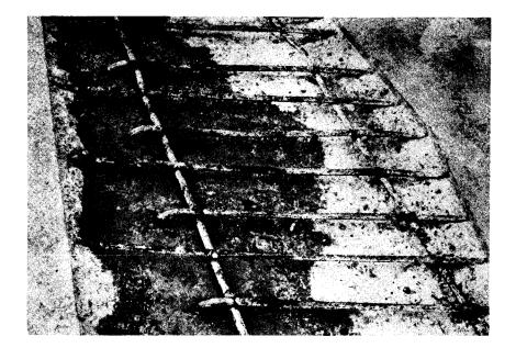
Figure 8. Close-up of reinforcement showing variable corrosion.
