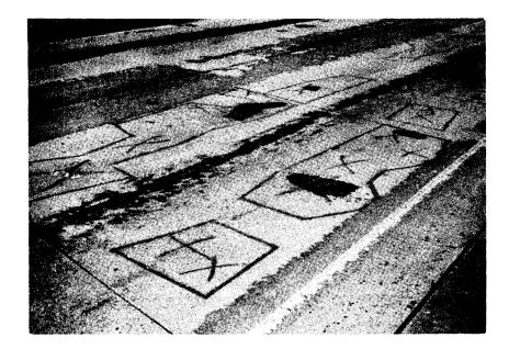
Figure 4. Area of moderate to severe spalling.
