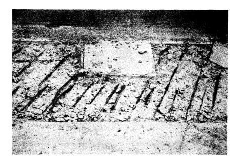
Figure 9. Area designated for repair adjacent to area repaired in 1970.
