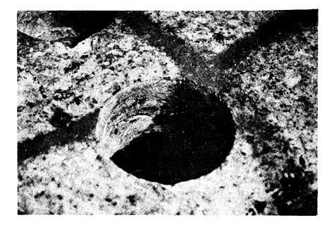
Figure 6. Close-up of incipient spall in Figure 5.
