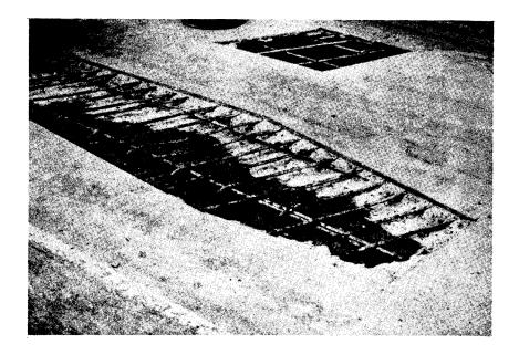
Figure 7. Large repair area.
